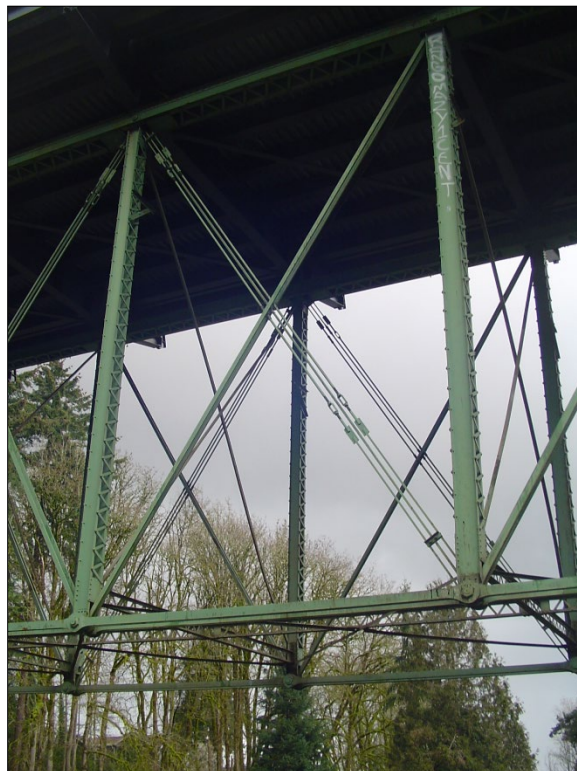
Photograph 8 of 12: OR_MultnomahCounty_BalchGulchBridge_0008 Detail view of 160' deck truss, center panel, looking north.
