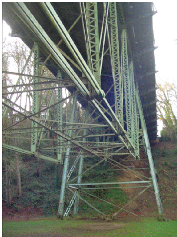
Photograph 6 of 12: OR_MultnomahCounty_BalchGulchBridge_0006 Underside of the Balch Gulch Bridge, looking west.
