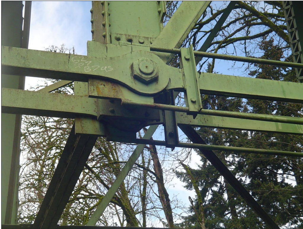
Photograph 11 of 12: OR_MultnomahCounty_BalchGulchBridge_0011 Detail of pin connection on 160' deck truss, looking north.
