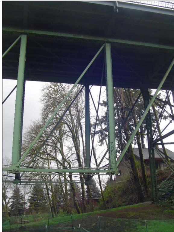
Photograph 9 of 12: OR_MultnomahCounty_BalchGulchBridge_0009 Southeast corner of 160' deck truss, looking north.
