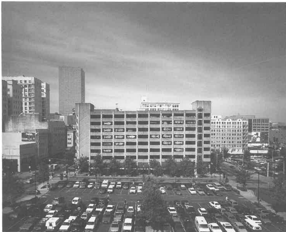
PARKING GARAGE - SW 3RD & ALDER
