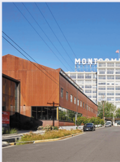
Development on NW Wilson which repurposed an existing industrial building with an updated form and new materials.
