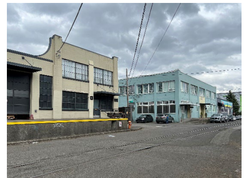
Existing dock conditions on NW York Street
