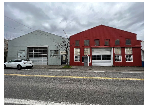
Existing industrial warehouses on NW Vaughn Street
