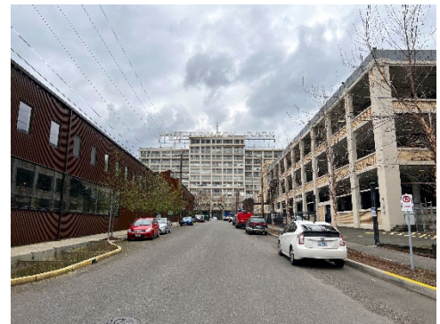
View of Montgomery Park and American Can
