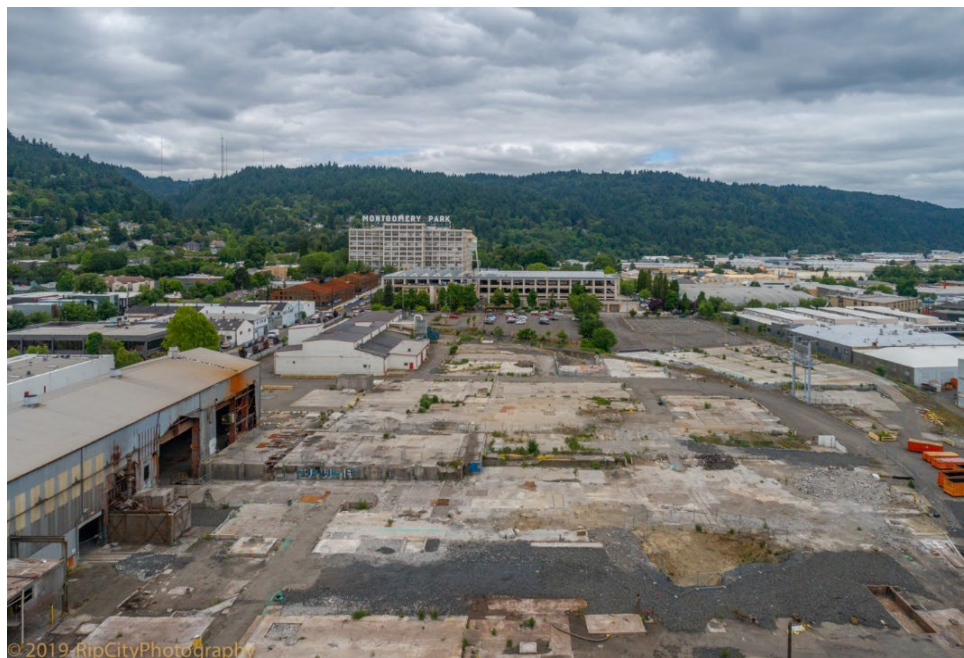
The former ESCO site (foreground) adjacent to Montgomery Park (background) is primarily vacant and is a redevelopment opportunity.
