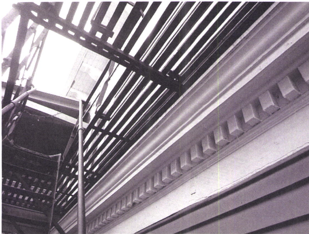
Missing diagonal compression strut. Decorative trimwork on wall directly under existing platform.
