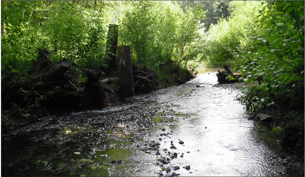
Tryon Creek sampling location #0208, at the restoration project near 4th Ave. The creek had eroded its banks and exposed a sewer pipe. The restoration project protected and stabilized the sewer pipe, and enhanced aquatic habitat by redirecting the creek away from the pipe, adding large wood, creating pool and riffle habitats, and revegetating riparian and floodplain areas.
