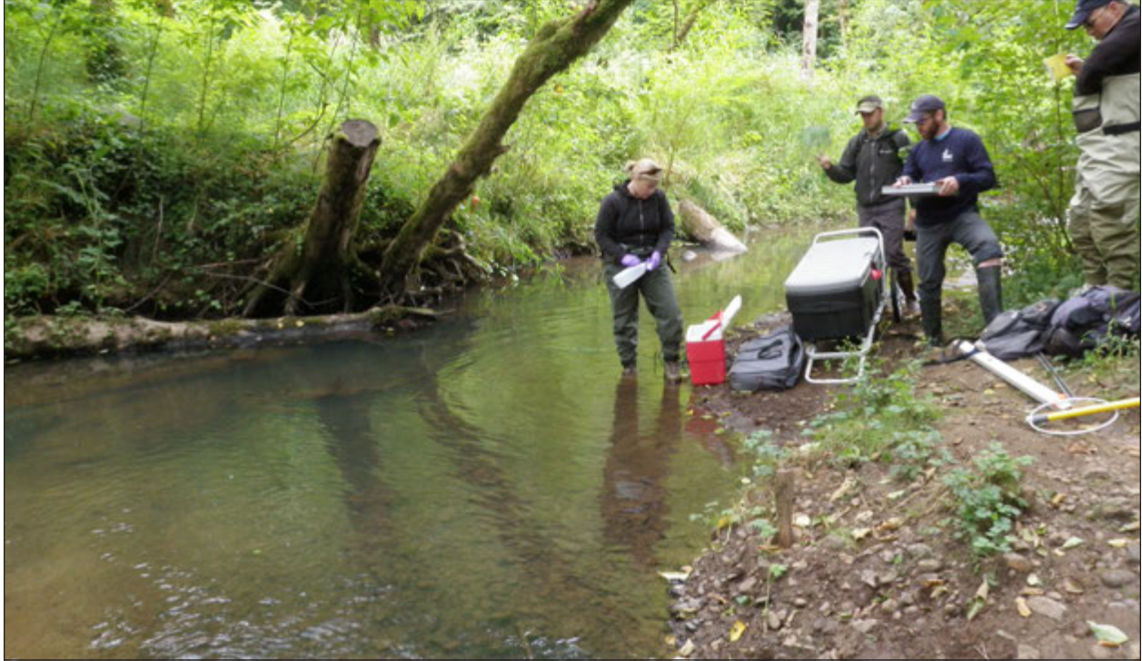
Tryon Creek sampling location #0208, at the restoration project near 4th Ave. The creek had eroded its banks and exposed a sewer pipe. The restoration project protected and stabilized the sewer pipe, and enhanced aquatic habitat by redirecting the creek away from the pipe, adding large wood, creating pool and riffle habitats, and revegetating riparian and floodplain areas.
