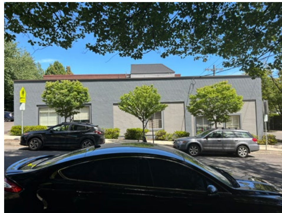
D) Porter Street Frontage - Facing North
