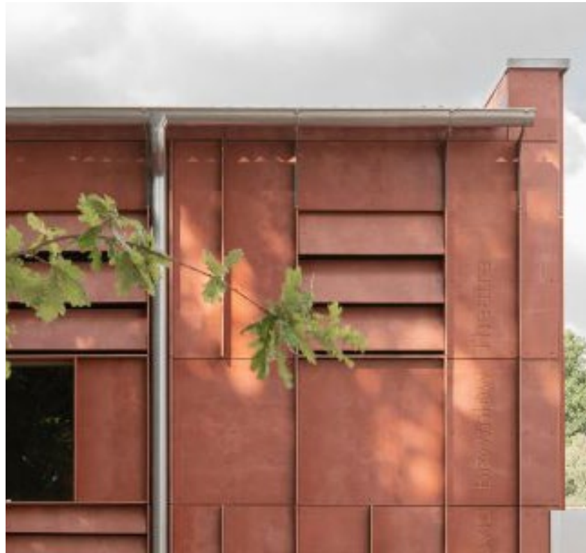
COMPOSITE WOOD FIBER AND CEMENT PANEL
