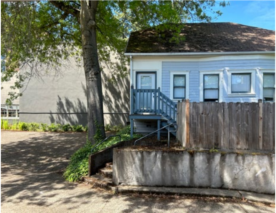
C) 118 SW Porter St - Facing West
