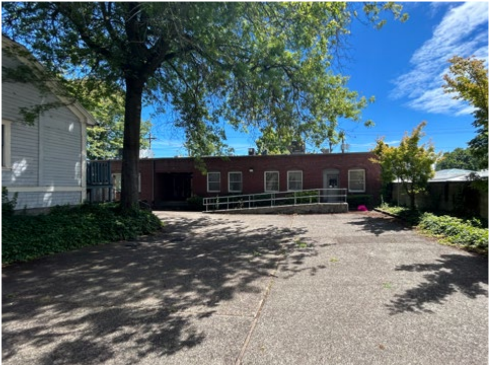
C) Existing on-site Parking - Facing East
