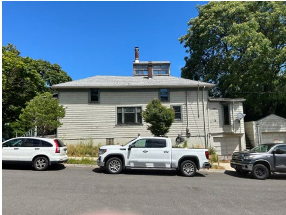
A) Porter Street Frontage - Facing North
