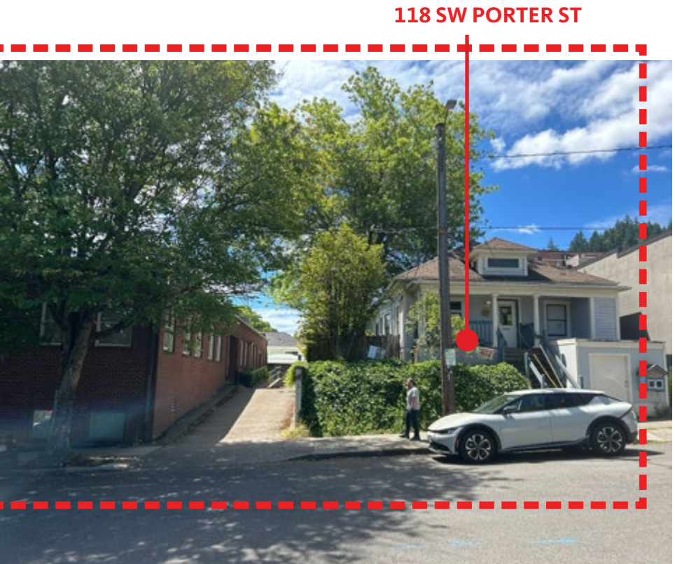
B) Porter Street Frontage - Facing South
