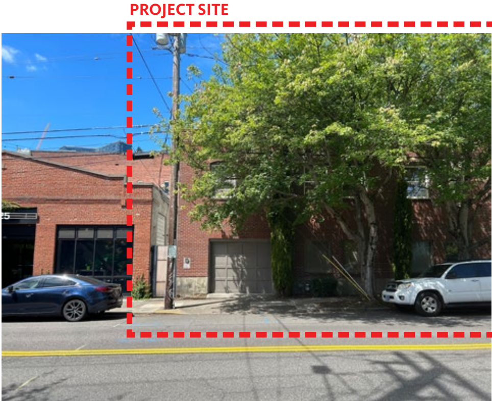
C) SW 1st Ave. Frontage - Facing West
