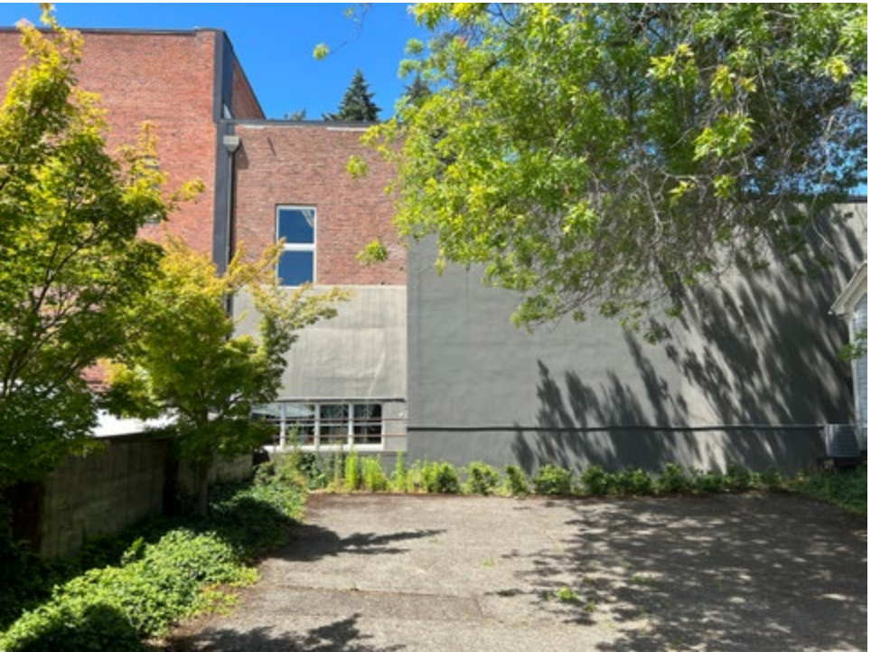
D) Existing on-site Parking - Facing West
