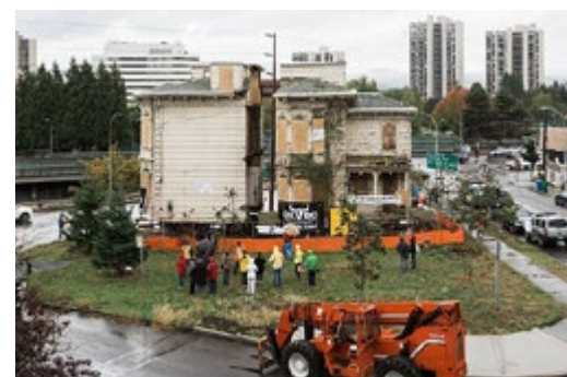
Photos of Fried-Durkheimer House relocation
