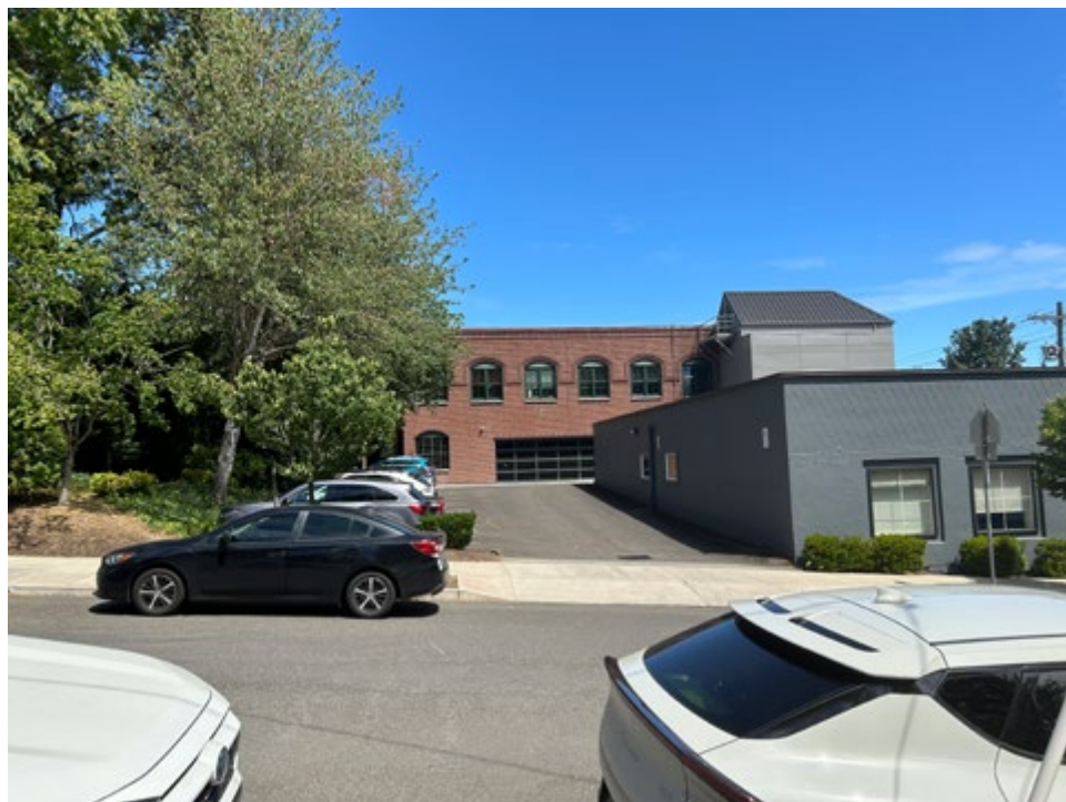
C) Porter Street Frontage - Facing North
