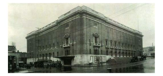
The late-1960s renovation was extensive and completely removed and rebuilt the interior, the front (west) façade, and the stage end (east) part of the building. However, the primary structural system holding up the roof, the masonry brick walls running east-to west along the north and south sides of the building, and the roof structure itself were not replaced and remain intact today.
