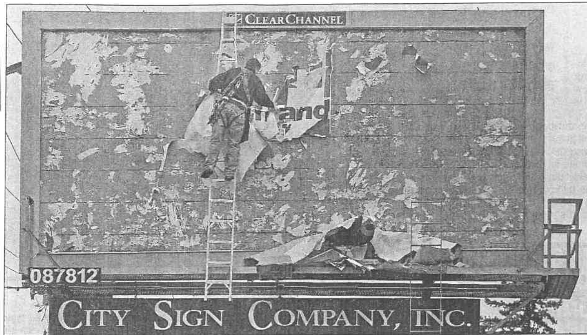
A worker from the City Sign Co. Inc. peels away an old billboard ad in preparation for applying a new one along Southeast Stark Street near 146th Avenue. TRIBUNE FILE PHOTO: L.E. BASKOW
