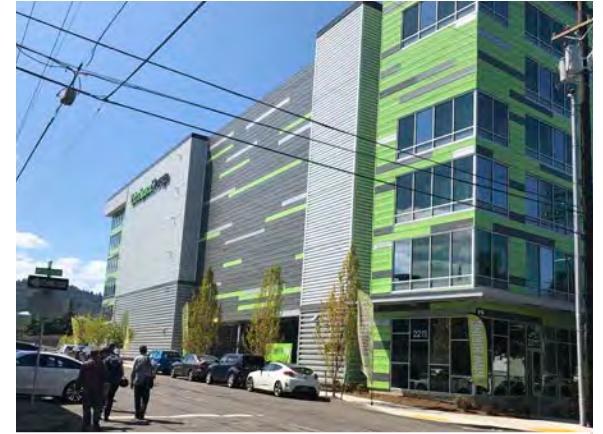
A newer building in the district housing storage units.
