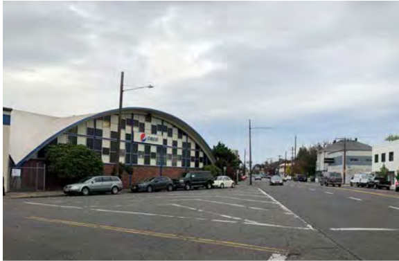
Large triangles of unused roadway space are a unique feature of the Sandy corridor, where the diagonal roadway crosses the typical street grid.
