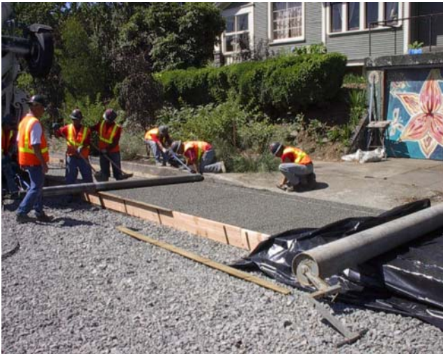
Figure 5: Laying the concrete
