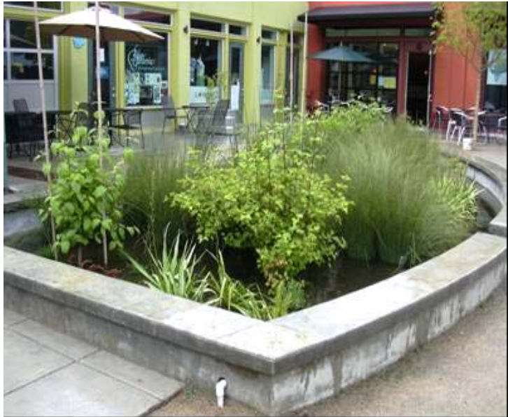
Stormwater Infiltration Planter, looking north
