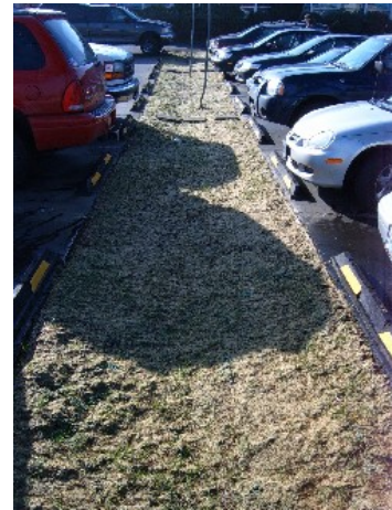
Figure 6: Jute mat and grass seed erosion control in repaired swale
