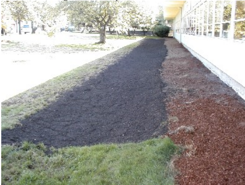
Figure 4: Grassy swale following construction
