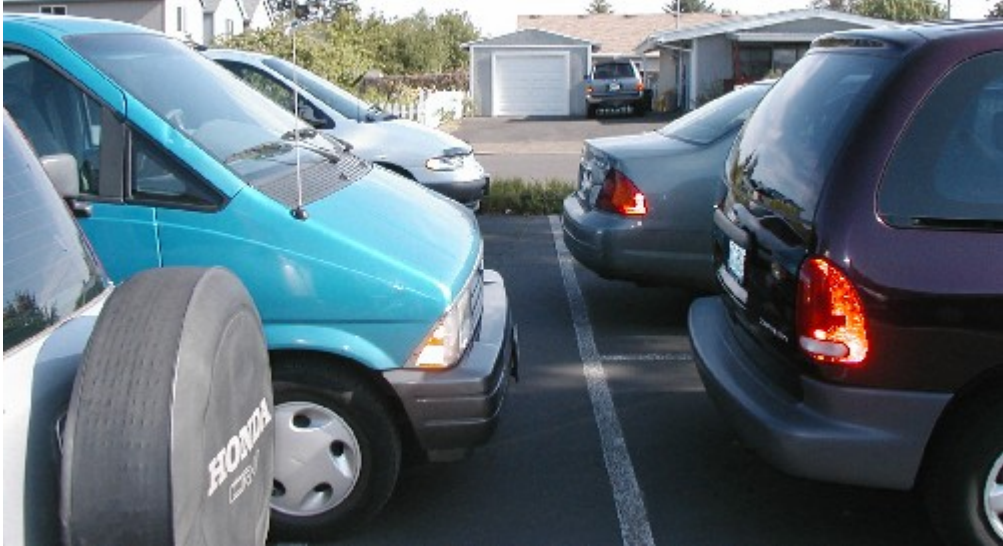
Figure 1: Asphalt between facing parking spaces
