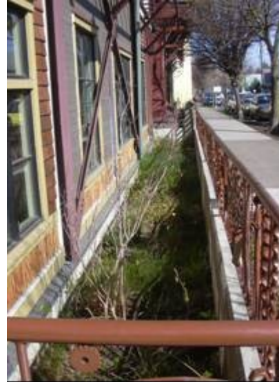
The flow-through planters in front of the new Mississippi Canopy with existing warehouse in the background
