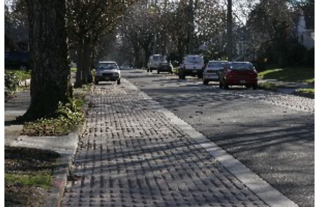
Figure 2: Pavers along parking strips only
