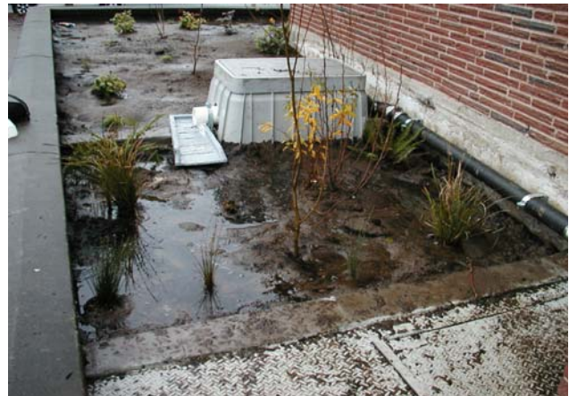
Figure 4: Installed monitoring equipment
