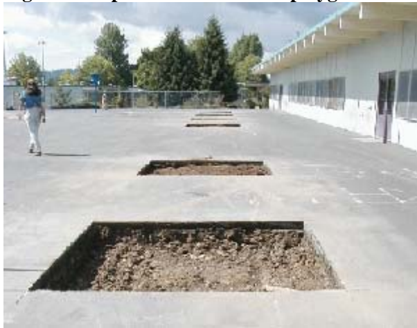
Figure 1: Asphalt removed from playground
