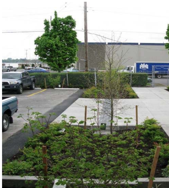
East facility after construction
