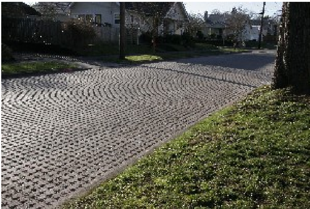
Figure 3: Pavers along the full length of the street
