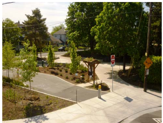
Looking east after construction
