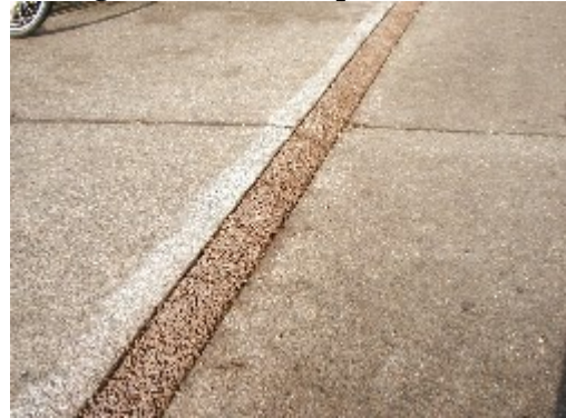
Figure 6: Porous asphalt radials
