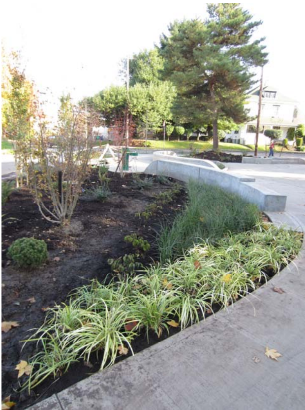
The infiltration basin accepts runoff from the plaza inside Holman Park. It has a 3:1 slope on all sides and a ponding depth of 6". In an overflow situation, water spills into the landscape area north of the facility.
