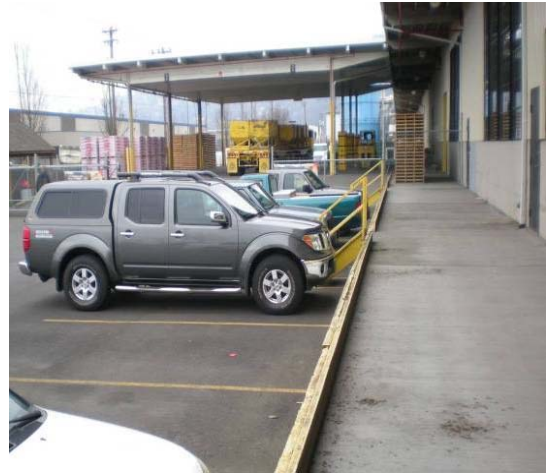
Loading dock before construction
