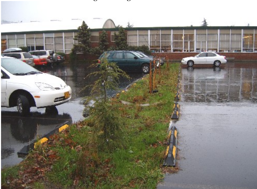
Figure 3: Vegetated swales
