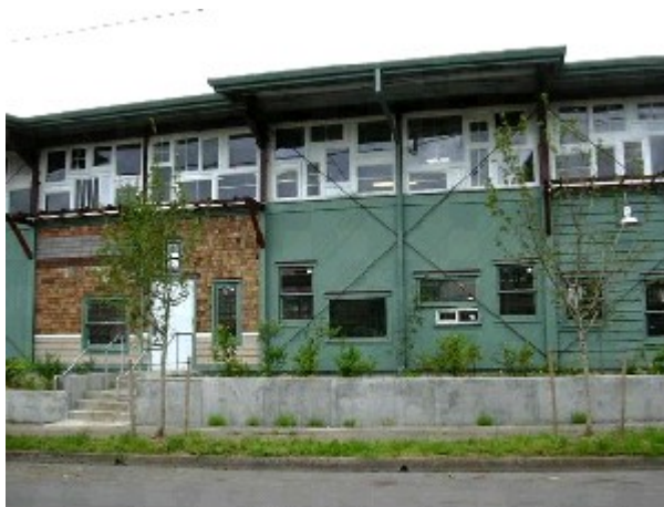
Infiltration planters along the Michigan canopy structure
