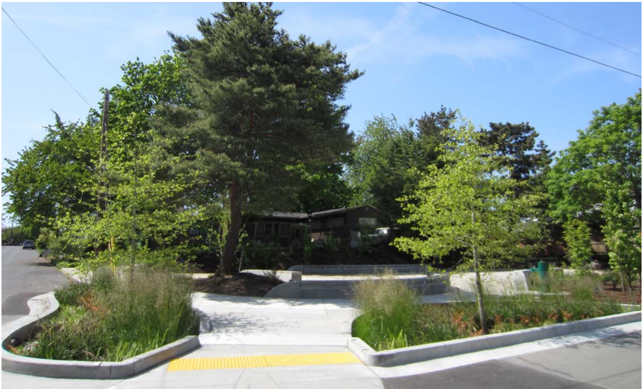
Two green streets in the ROW adjacent to the park accept runoff from the street. They are flat bottom infiltration facilities with a ponding depth of 6". Water enters the first facility (left), ponds to 6", then enters the second facility (right) by way of a trench grate. An emergency overflow beehive inlet in the second facility directs water to a sedimentation manhole and sump.
