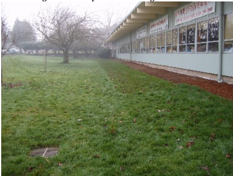
Figure 4: Grassy swale following construction
