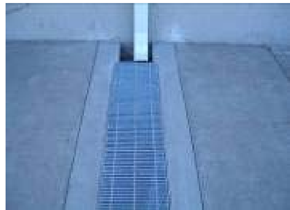
Runnel on loading dock
