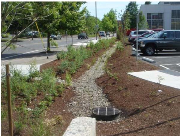
Vegetated infiltration swales east side of site post construction
