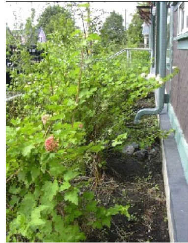
A downspout disconnected into the infiltration planters on Michigan Street
