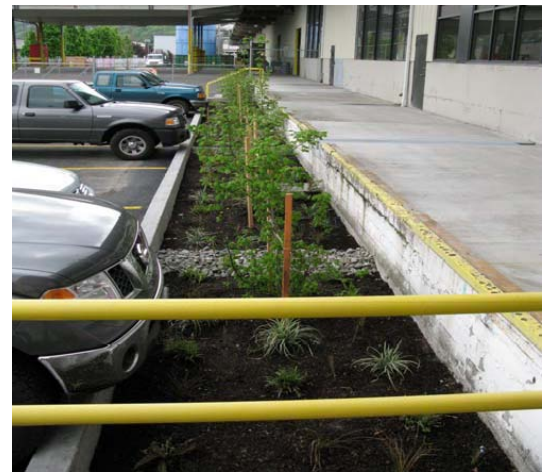
Loading dock after construction
