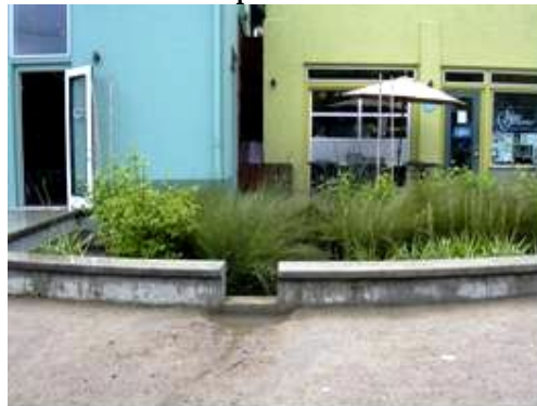
Roof runoff conveyed to the newly vegetated planter
