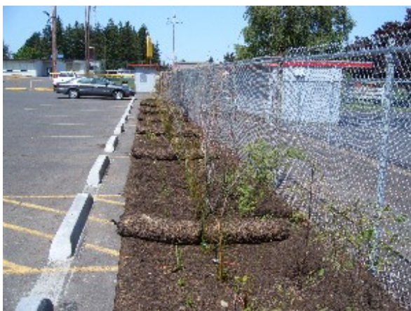
Figure 3 – east swale post construction
