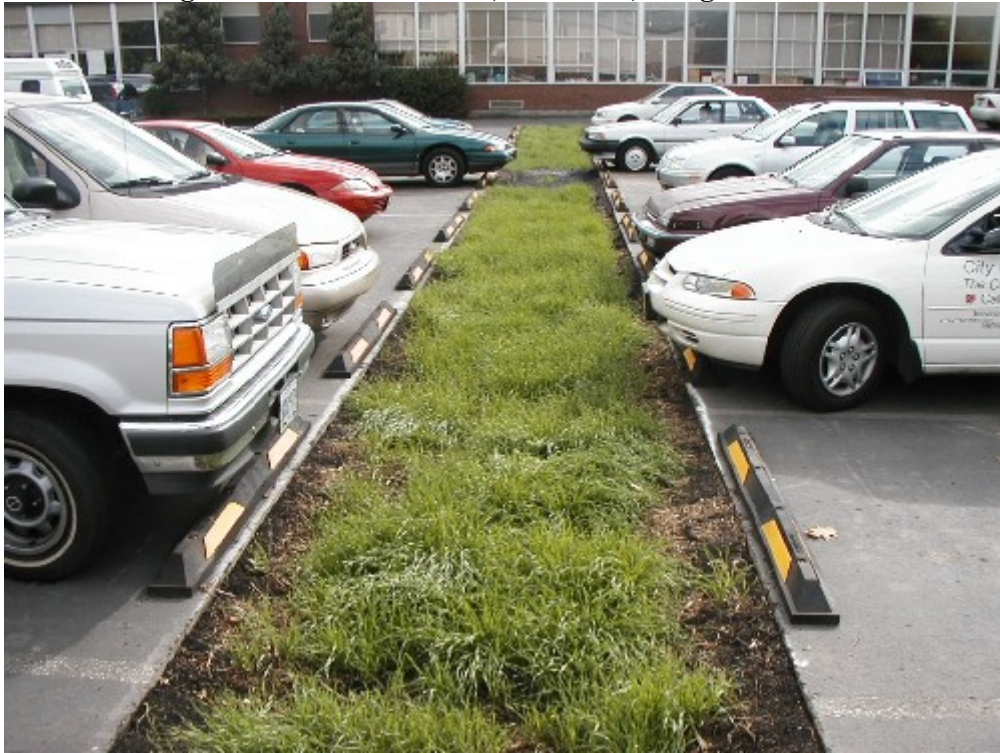
Figure 2: Swales excavated, backfilled, and grass seeded
