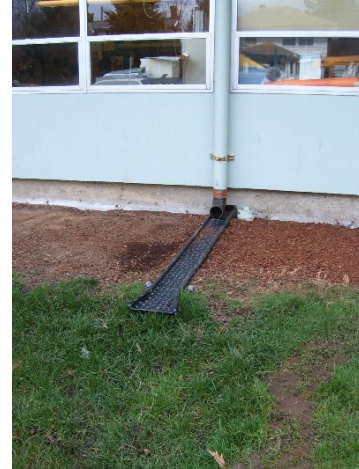
Figure 5: Downspouts disconnected to grassy swale
