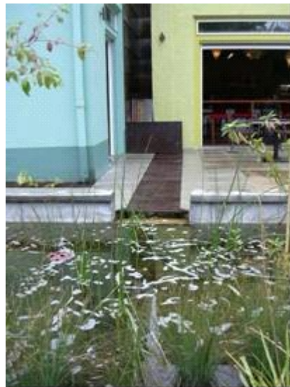
Roof runoff conveyed to the newly vegetated planter
