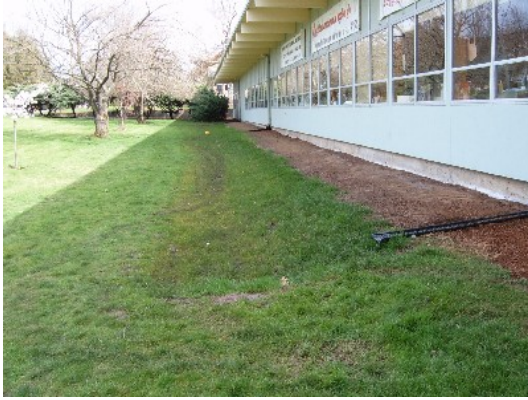
Figure 5: Downspouts disconnected to grassy swale
