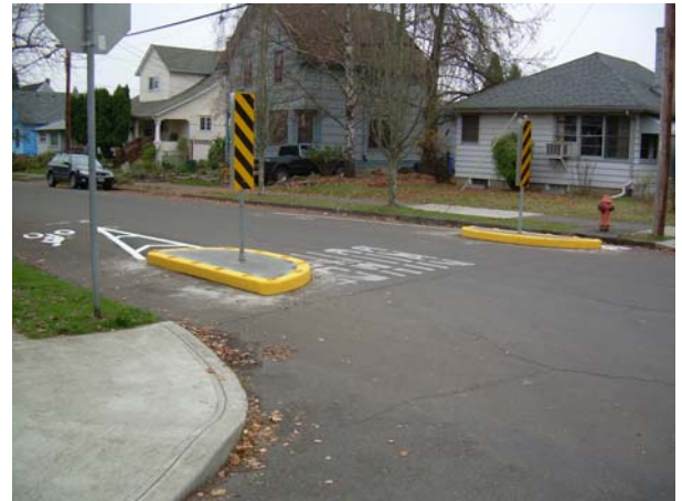
Channelizer Island at SE 15 th Avenue
