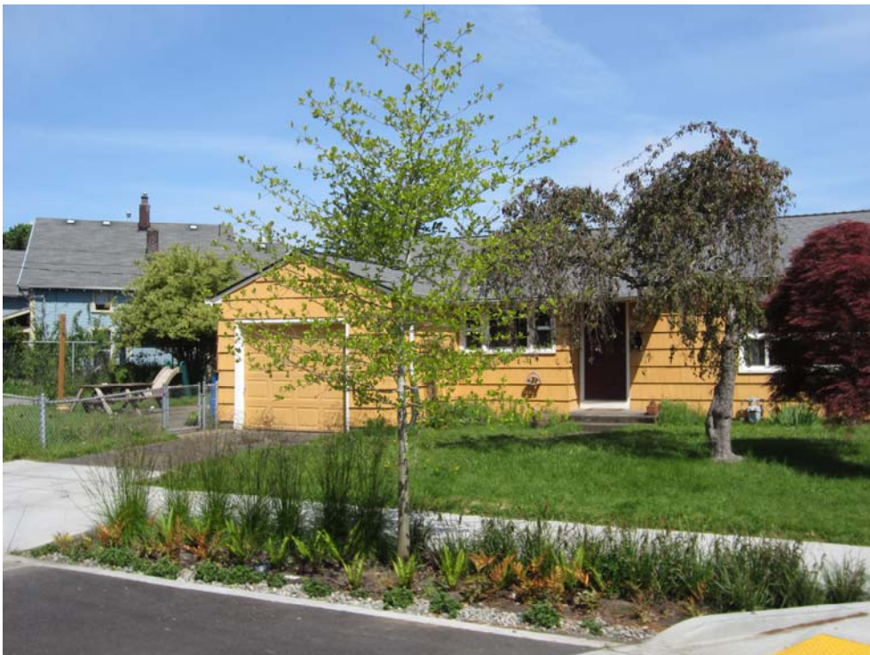
Two filter strips were constructed in the ROW north of the park. They are flat bottom infiltration facilities with a 3" ponding depth. Water enters from the street over the flush curb. The emergency overflow runs back into the street and to a catch basin east of the site where the water previously drained.
