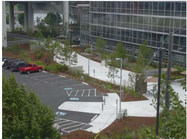
Clay Street from above looking east post-construction
