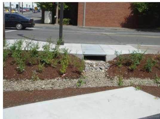
Public to private inlet at Water Street
