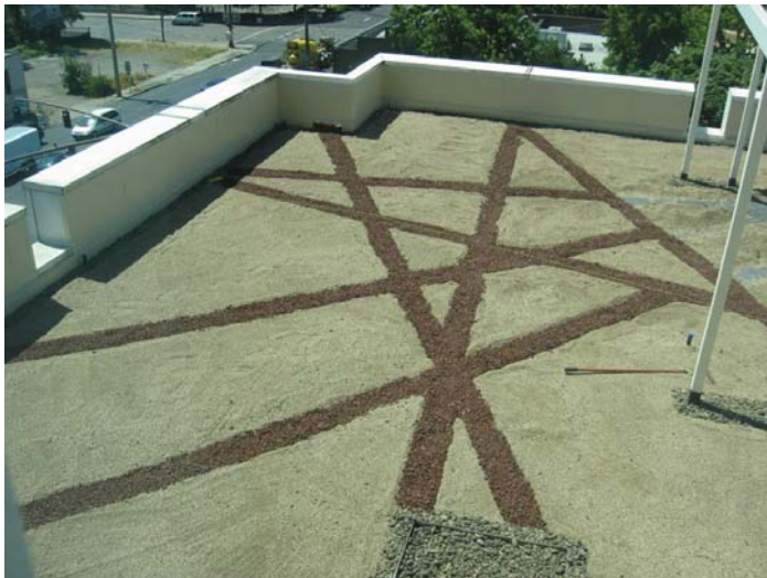
Cinder Rock Drainage Channels
