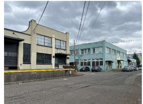
Existing dock conditions on NW York Street
