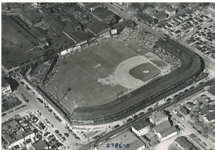
Vaugh Street Park, 1951
