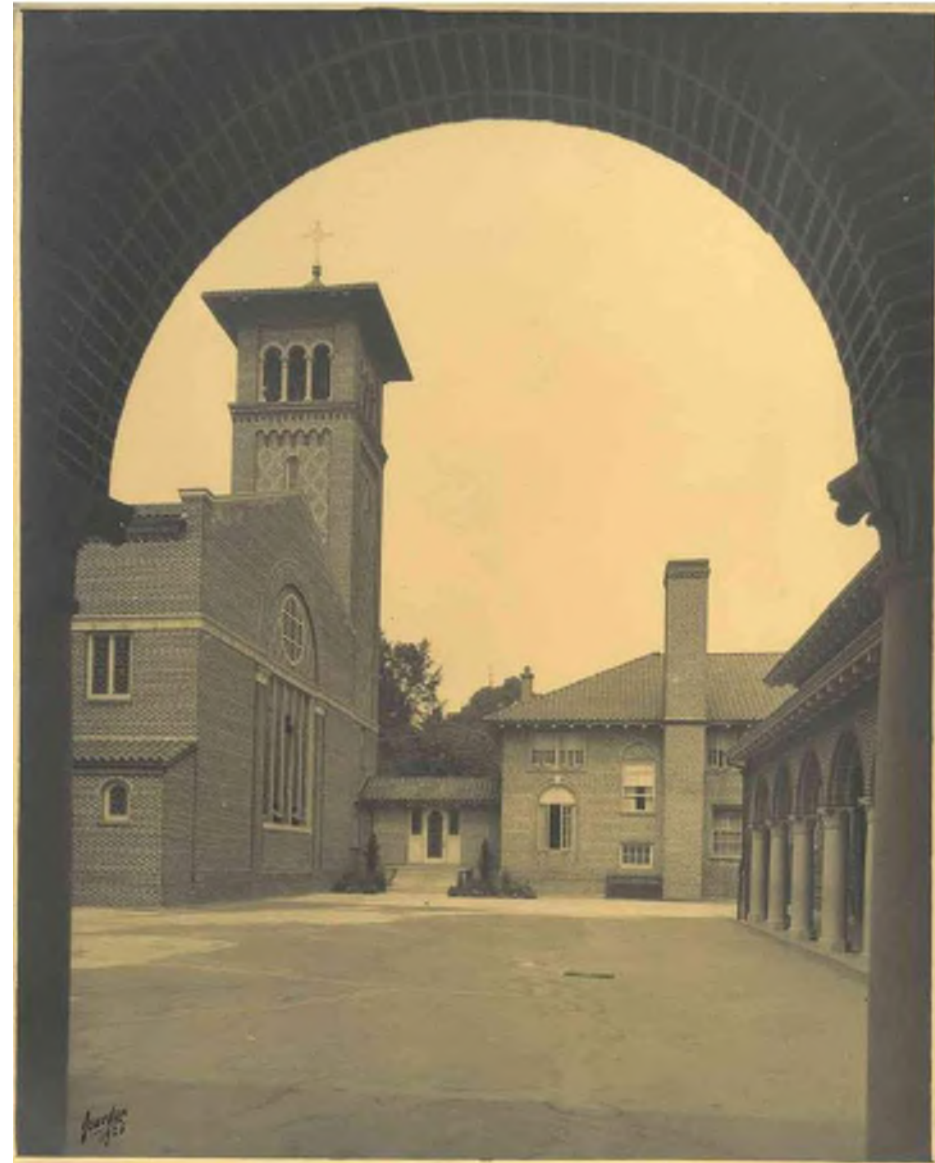
FACING NORTH INTO THE COURTYARD - 1926
