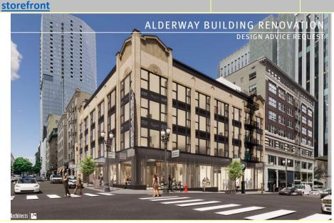
Proposal is to replace all existing ground floor cladding and glazing with a new structural silicone glazing system on a low stone base, replace existing fabric awnings with new metal canopies at entries and add new signage and exterior lighting. Proposal also includes a small new rooftop terrace/ amenity space.
