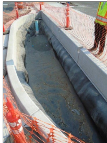
Fully-lined system with underdrain visible, just prior to loading blended soil
