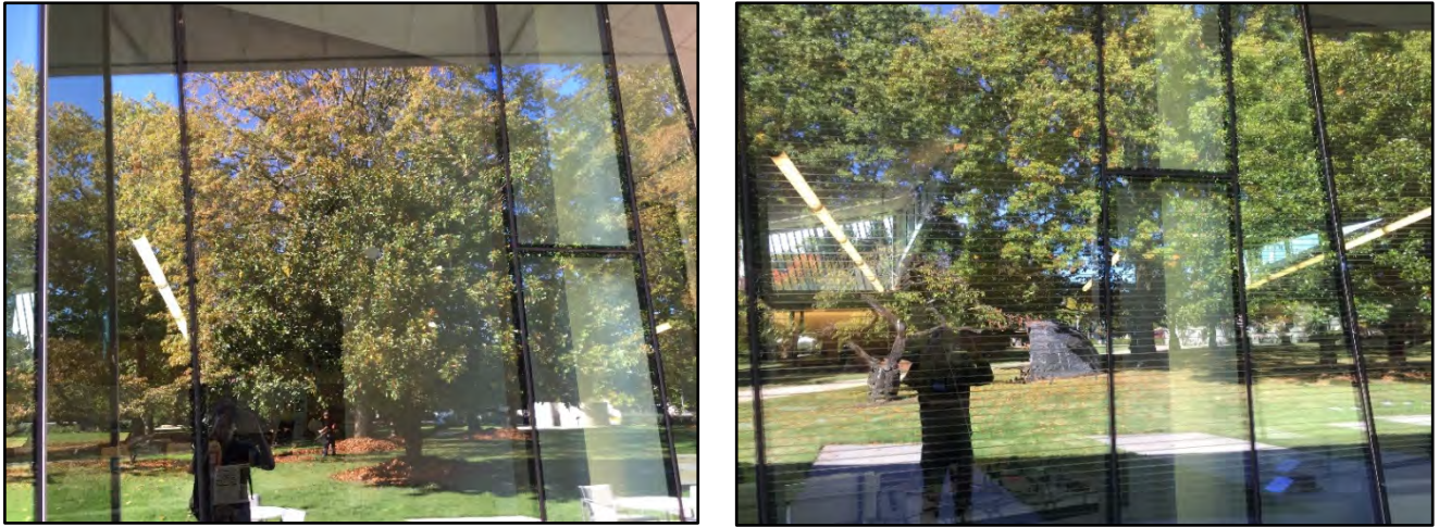
Photos 12 and 13: Windowpanes before (left) and after treatment retrofit (right)
