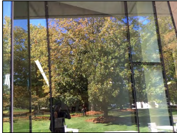
Photo 4: Example of the reflection hazard created by north facing windows adjacent to vegetated campus setting.
