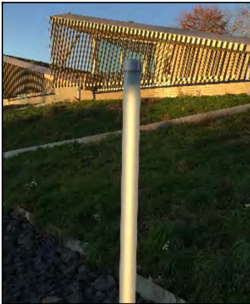
Photo 1: Example of unshielded tube light at the Columbia Building.
