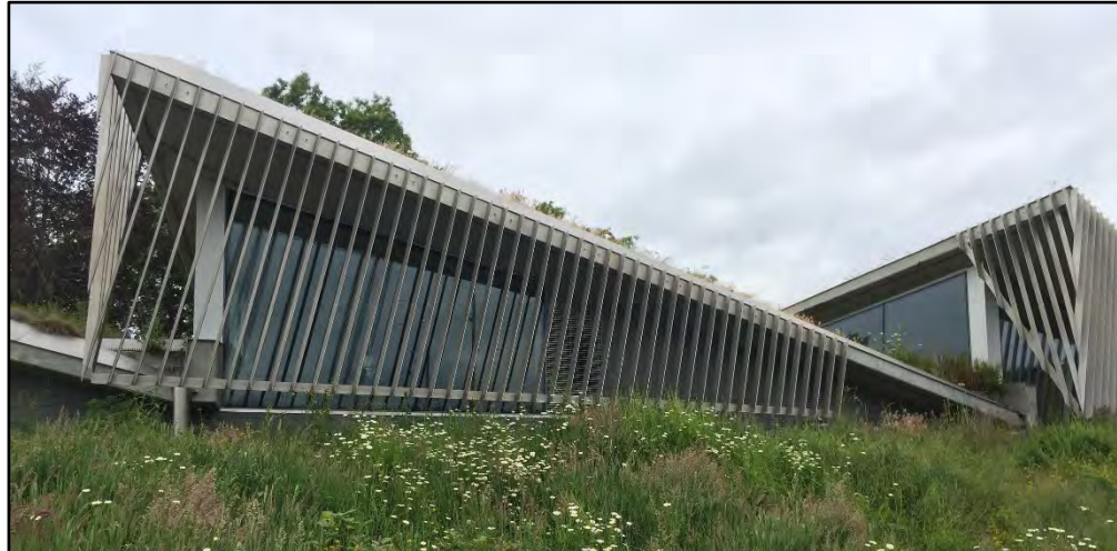
Photo 9: South facing window behind louvers. The triangular window on the right without louvers is one of the clerestory windows that faces the ecoroofs.
