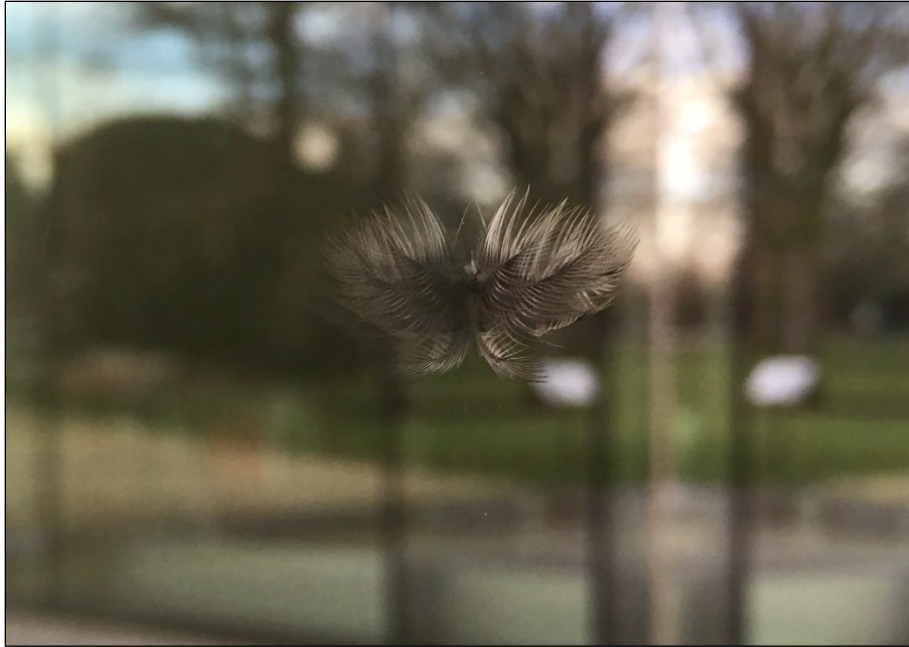
Example of feather evidence of a bird window strike at the Columbia Building north lobby windows. This feather is about 1 cm wide.
