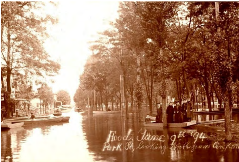
Figure 2: 1894 flooding along the North Park blocks (Portland Archives)
