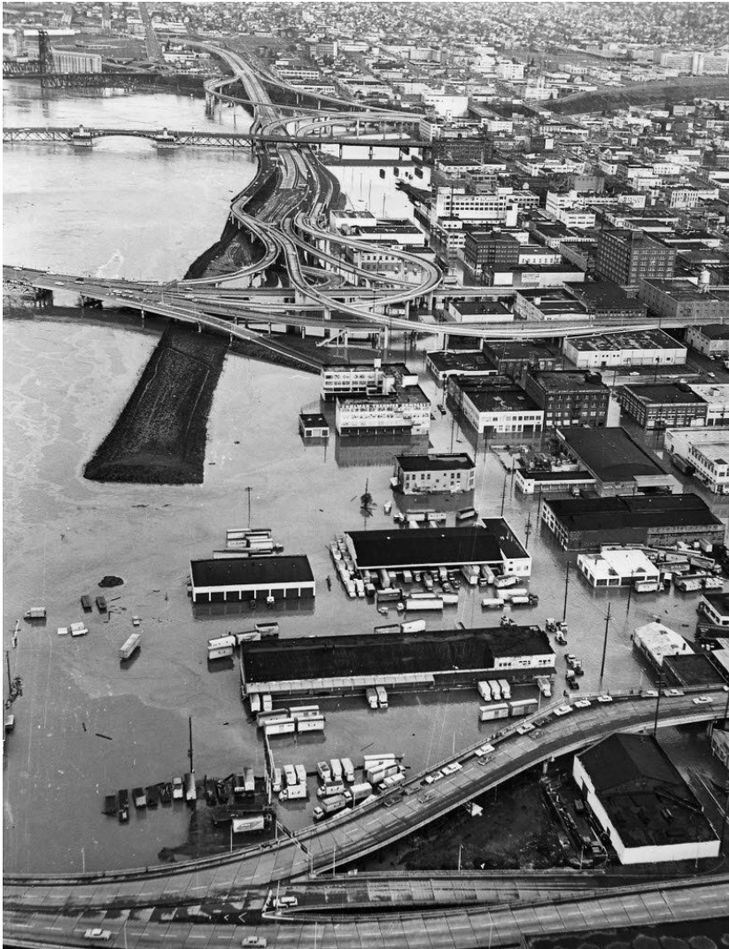
Figure 5: 1964 flooding of the Central Eastside (Credit: John Killen, The Oregonian )
