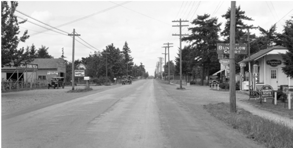
A 1934 photo showing SE 82nd Avenue (near SE Flavel St) with center strip paving and dirt shoulders and sidewalks
