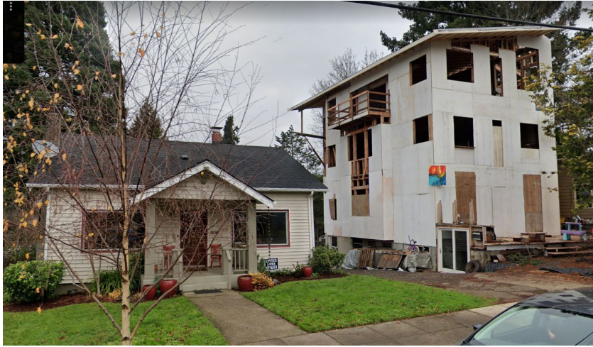
Pre-RIP house remodel
