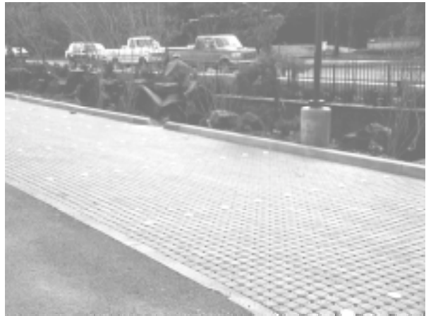
Pervious paving surface, Washington County, Oregon
