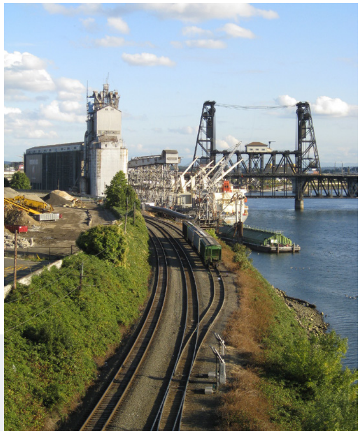
Image of the Willamette River waterfront hosting rail, marine freight, and grain elevators, with the Steel Bridge towering in the background. [Source: Chris Yunker]
