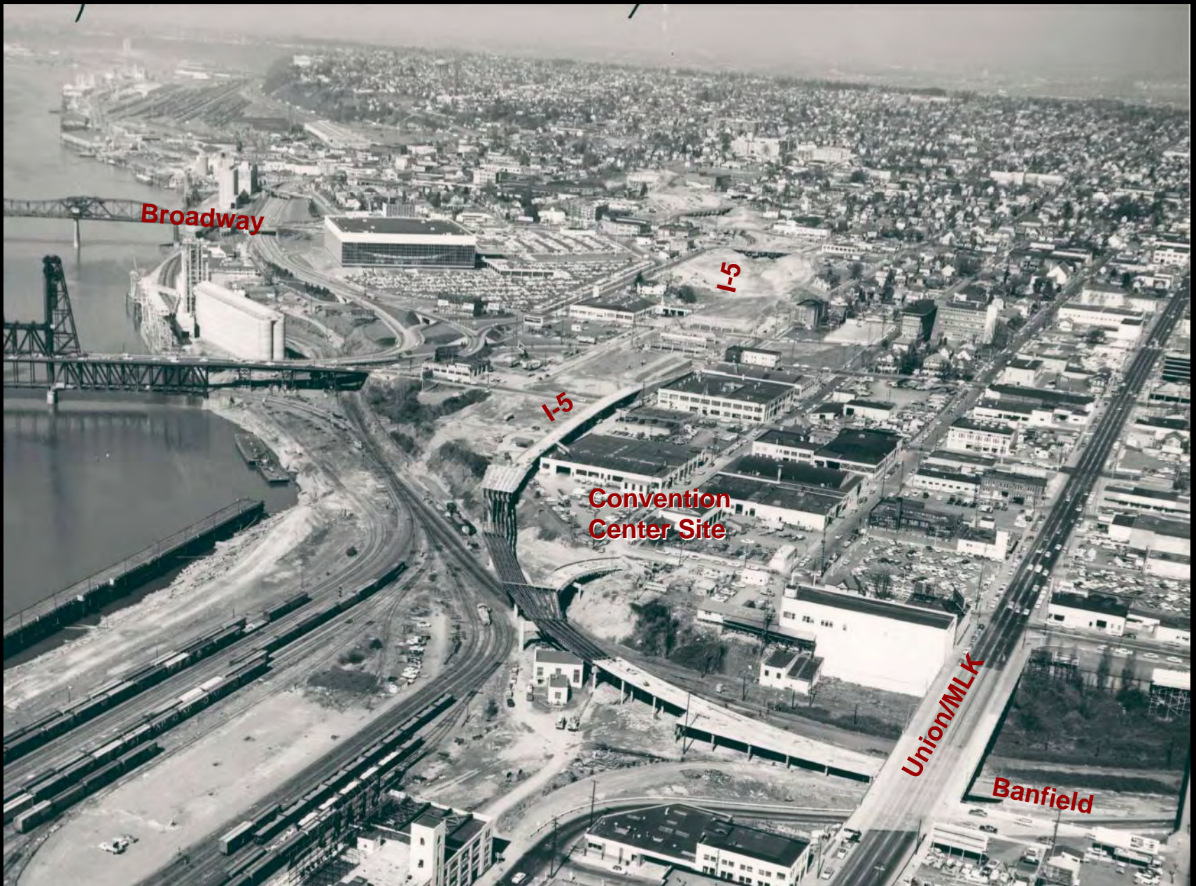
I-5 Construction at the I-84 Interchange, 1962
