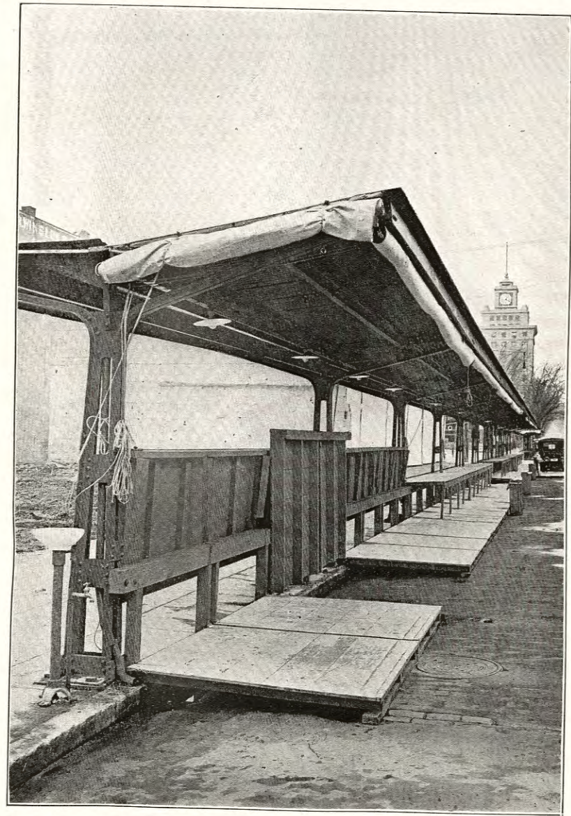
SECTION OF MARKET SHED, SHOWING METHOD OF RAISING TABLES AND FLOORS TO PROVIDE UNOBSTRUCTED STREET FOR FLOOR FLUSHING
