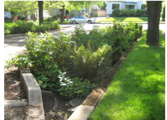
This street planter collects and treats stormwater onsite before filtering it back into the ground. Portland has 475 green streets to date, with 950 planned for the next five years.
