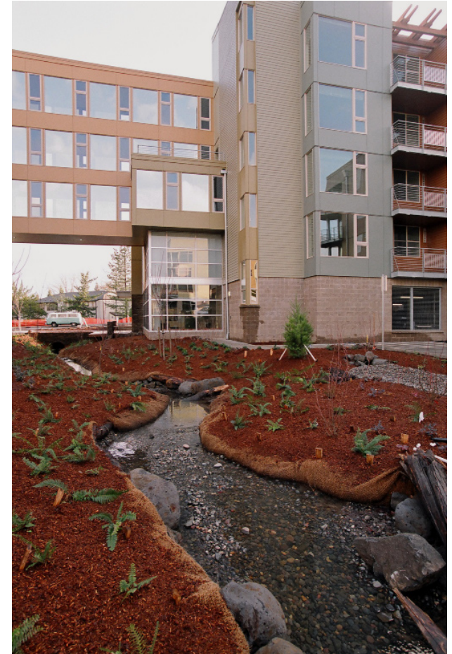
The new Village at the Headwaters, an affordable senior apartment community in Southwest Portland, designs within an environmental watershed context by “daylighting” an existing stream and incorporating swales and rain gardens for stormwater management. Such sustainable features create and enhance value for the property and its residents.
