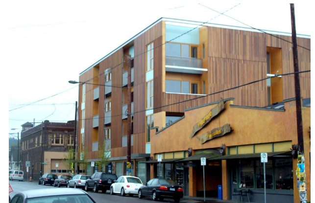
The emphasis both the City and Metro have placed on focusing development and density along corridors has resulted in larger condo developments such as this one on SE Belmont.
