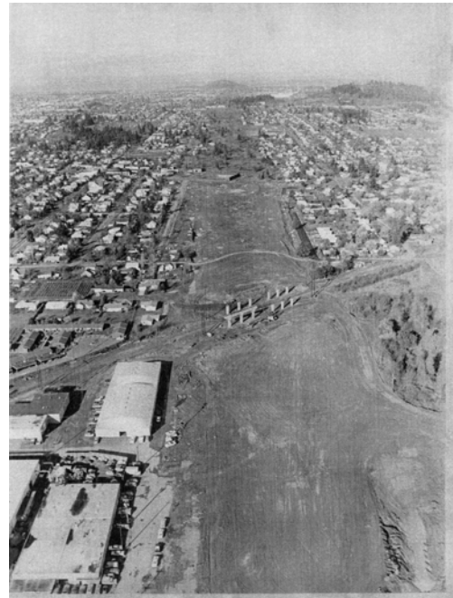
Construction of Interstate 205.
