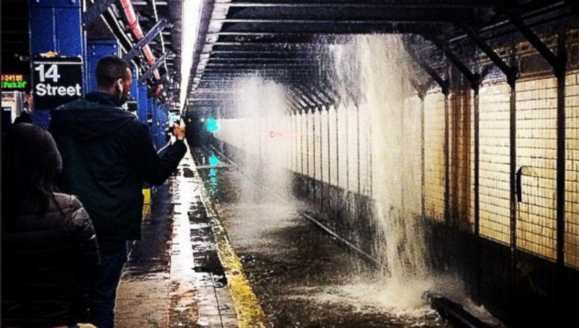
Rainwater flooding MTA New York City, 2018 (johnvlahakis/Instagram)
