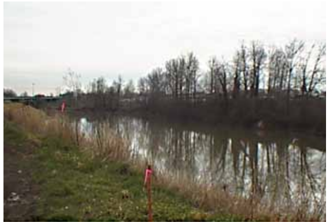
COLUMBIA SLOUGH AND LEVEE
