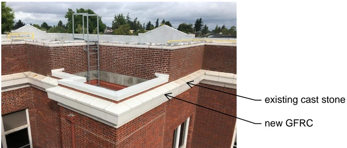
fig. 26: GFRC installed at Rose City Park Elementary
