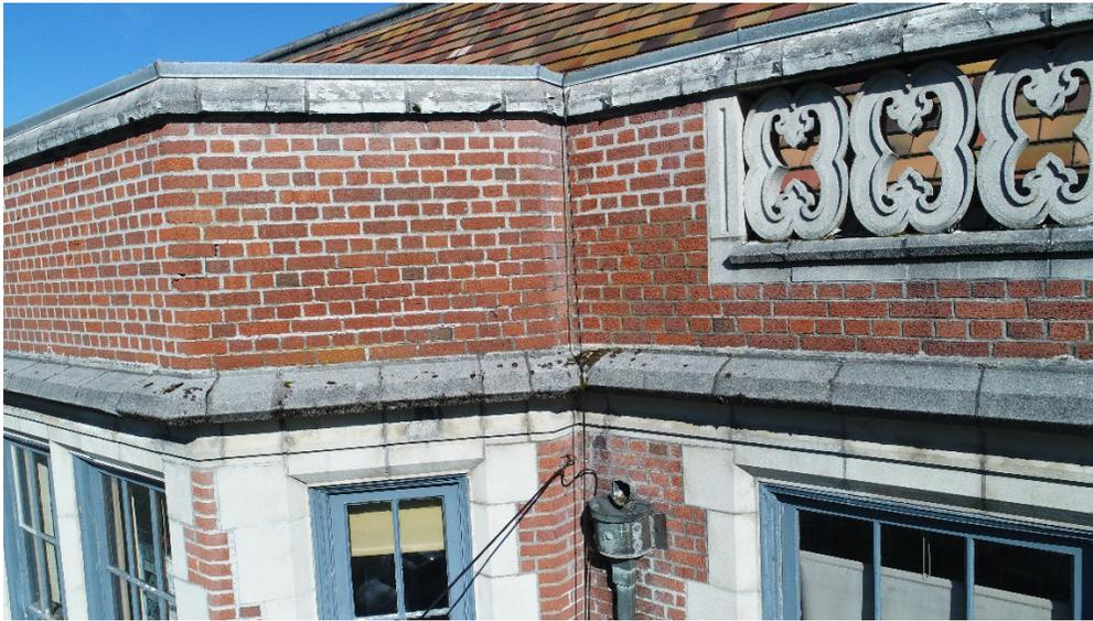
*Figure 9. Scupper, collection box, and downspout*
