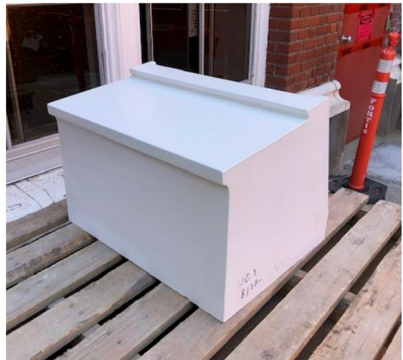
fig. 27: GFRC unit before installation
