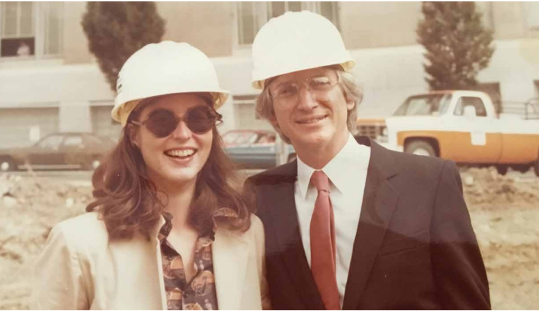
Michael Graves (right) and Lisa Lee Morgan (left) at the Portland Building site during construction circa 1980.
