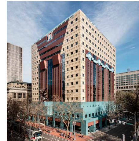
(left to right) The Portland Building soon after completion in 1983, pre-reconstruction in 2016, under construction in 2018 and after reconstruction in 2020.
