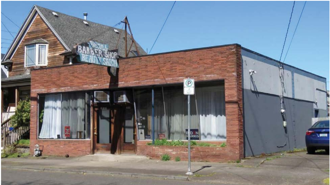
Dean's Barbershop, Listed to the National Register of Historic Places in 2022. Photo Credit: National Park Service
