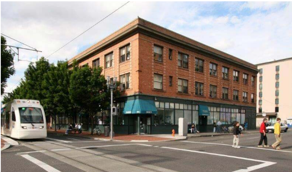
Central City Concern's Medford Hotel, which comprises 61 SRO units. It is a URM building.
