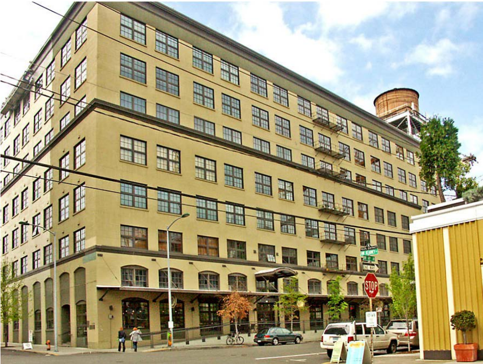
The Marshall Wells Lofts project in the Pearl District converted a 1910 warehouse into condos, taking advantage of the State Special Assessment Program that provided condo owners with a 10-year property tax freeze, making them more affordable.
