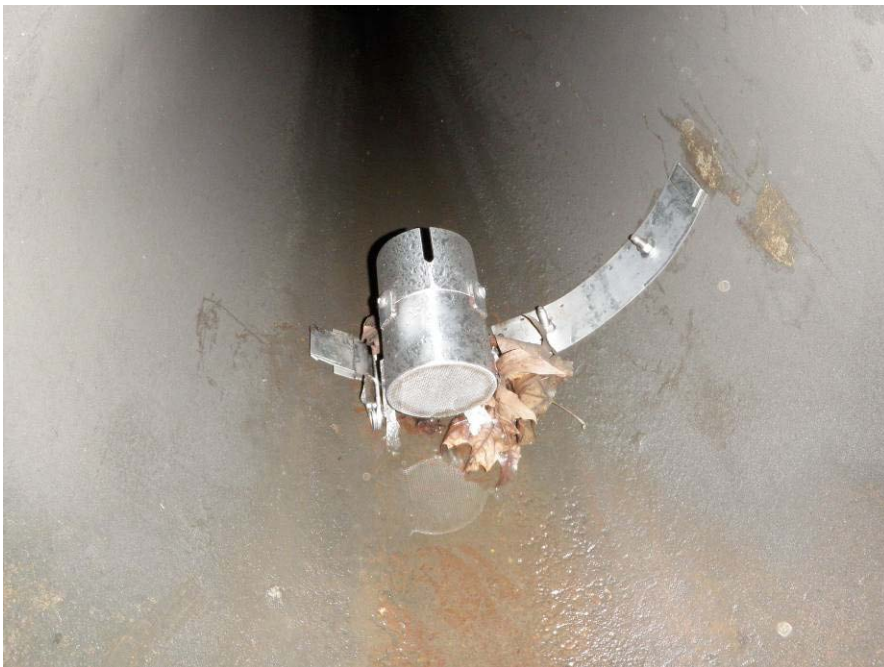
Photo 2 (March 17, 2010). Screened Inline Flow-Through (SIFT)© 1 style sediment trap installed in the 21-inch line entering manhole AAM127 from the northwest.
