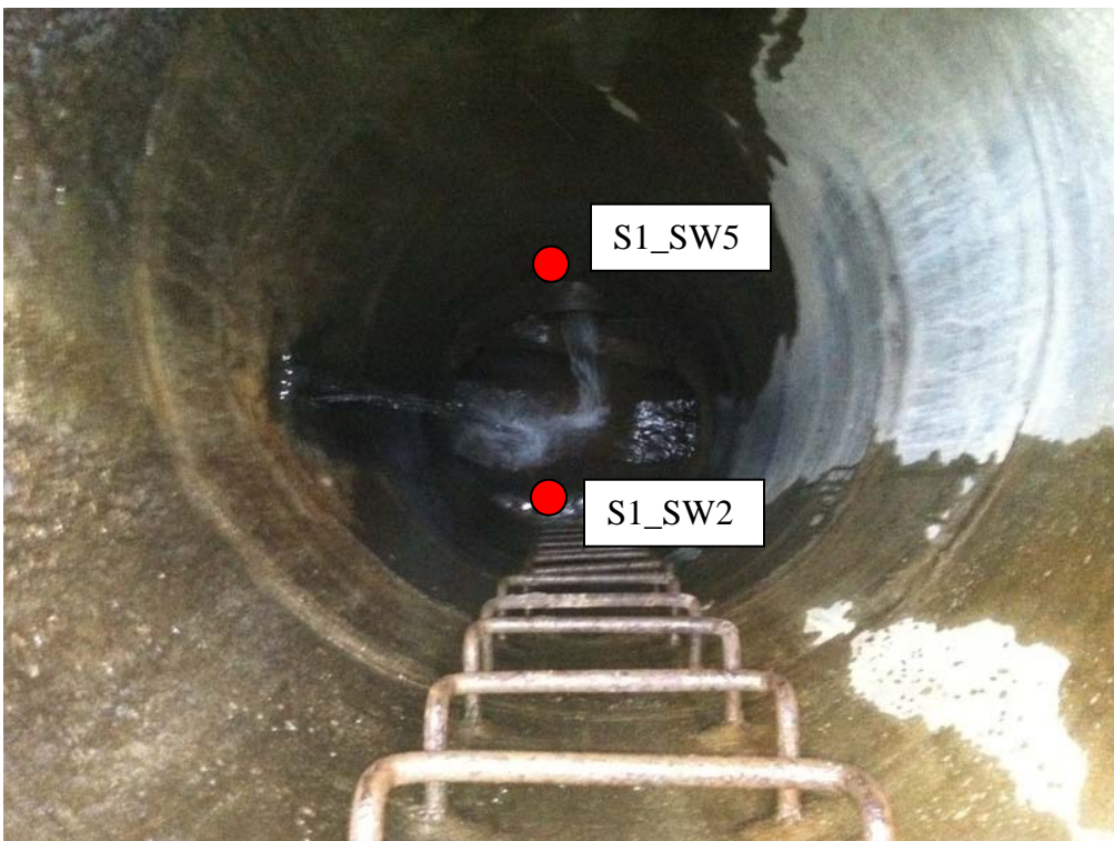
Photo 16 (April 14, 2011). View into manhole AAM127. Incoming 21-inch line from Shipyard site (SW5) and outgoing 27-inch line (SW2) are labeled.
