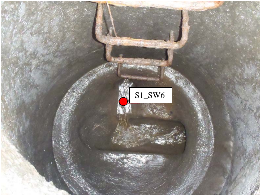
Photo 20 (April 28, 2011). View into manhole AAM138. Flow from incoming lateral from DSU Peterbilt site (SW6) is labeled.
