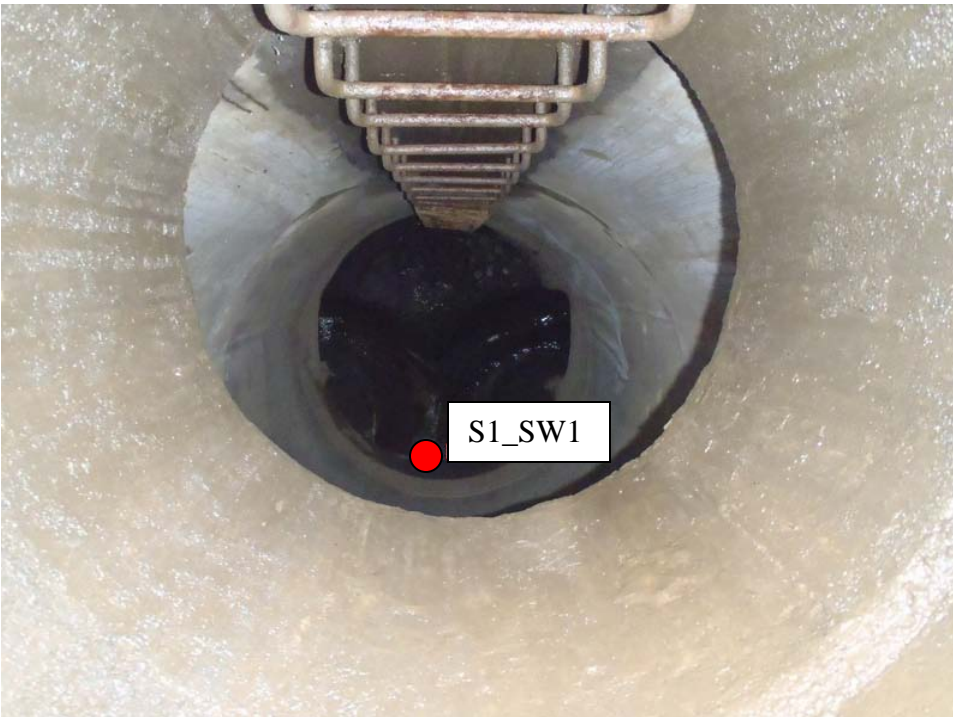
Photo 14 (April 28, 2011). View into manhole AAM131. Outgoing 36-inch pipe (SW1) is labeled.
