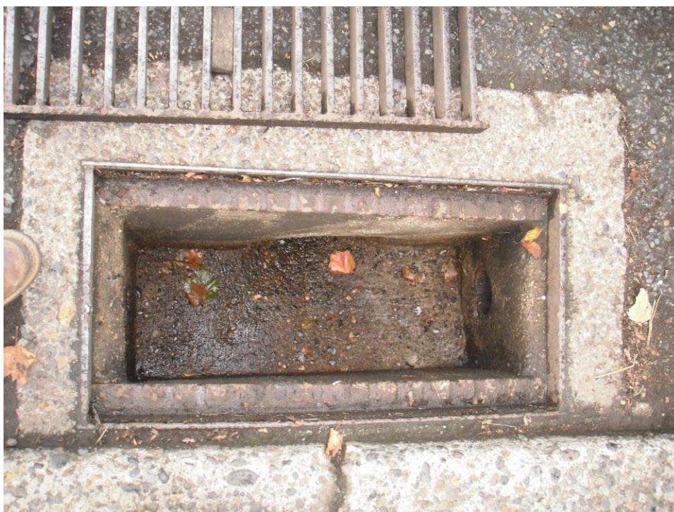
Photo 10. Catch basin ANE509; view of solids sampled.
