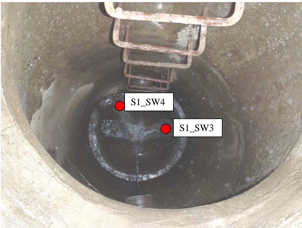
Photo 18 (May 11, 2011). View into manhole AAM133; incoming 15-inch lateral from EWH LLC site (SW4) and outgoing 18-inch pipe (SW3) are labeled.
