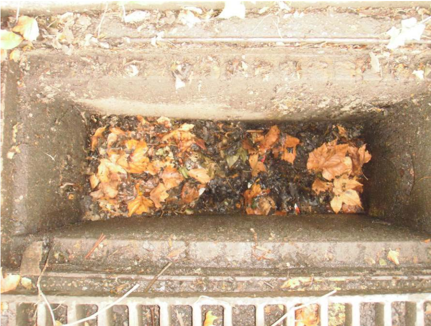
Photo 12. Catch basin ANE512; view of solids sampled.
