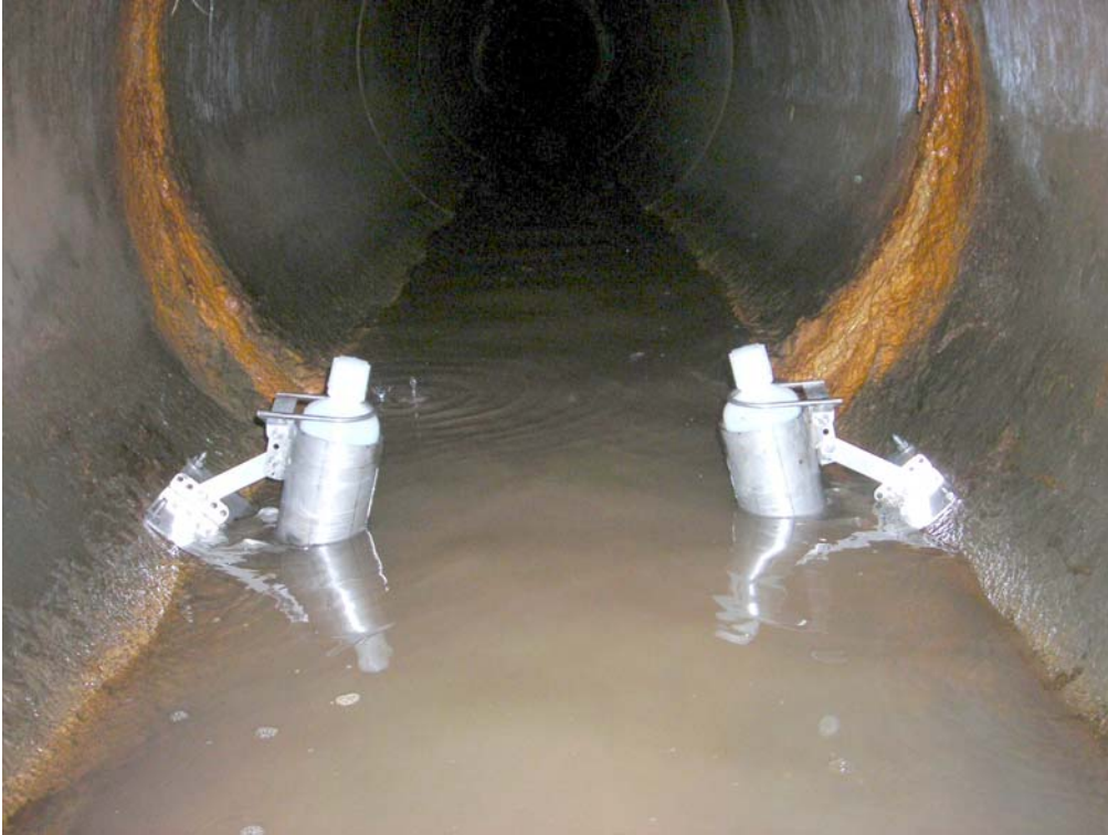
Photo 1 (March 2007). Sediment trap installation downstream of manhole AAJ994, looking downstream.
