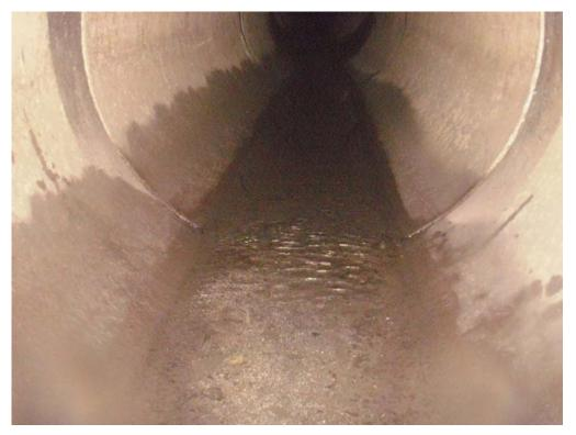
**Photo 17 (December 22, 2010):** Solids sampling location in 36-inch-diameter line discharging to Manhole AAA188.
