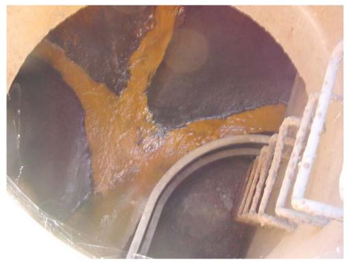
**Photo 5:** Looking into Manhole AAA179; discharges from the three laterals are apparent in this photograph.
