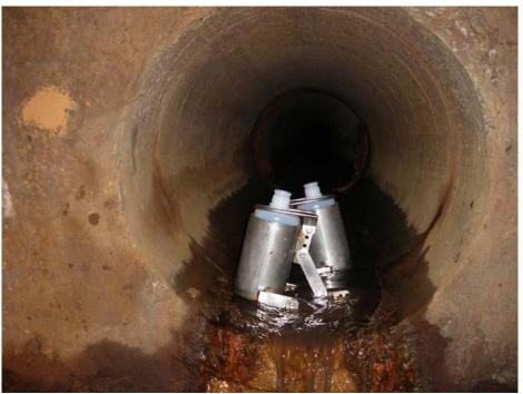
**Photo 8 (October 15, 2007)**: Deployed sediment traps at sampling location ST3; upstream of Manhole AAA179 in eastern branch.
