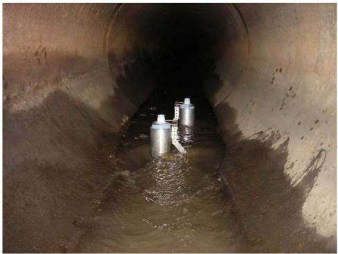
**Photo 11 (October 15, 2007):** Deployed sediment traps at sampling location ST4; upstream of Manhole AAA179 in southern branch.
