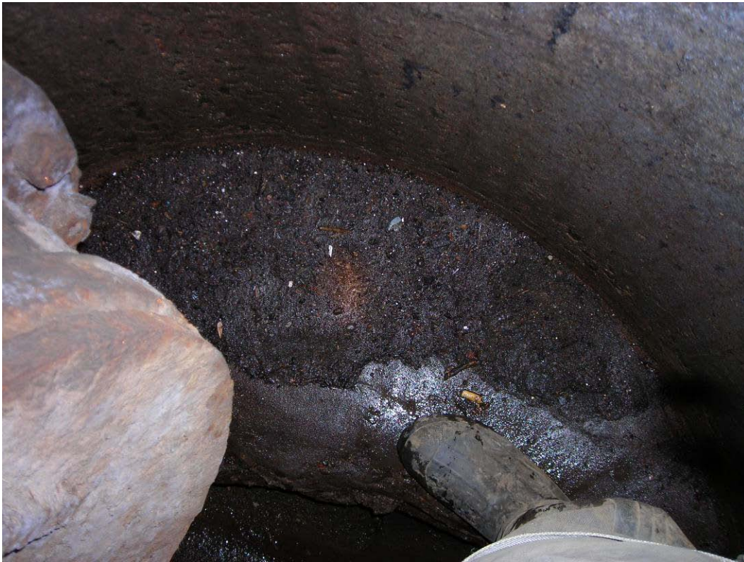
Photo 1 (June 26, 2008). View of solids accumulated on the eastern ledge in manhole AAE513.
