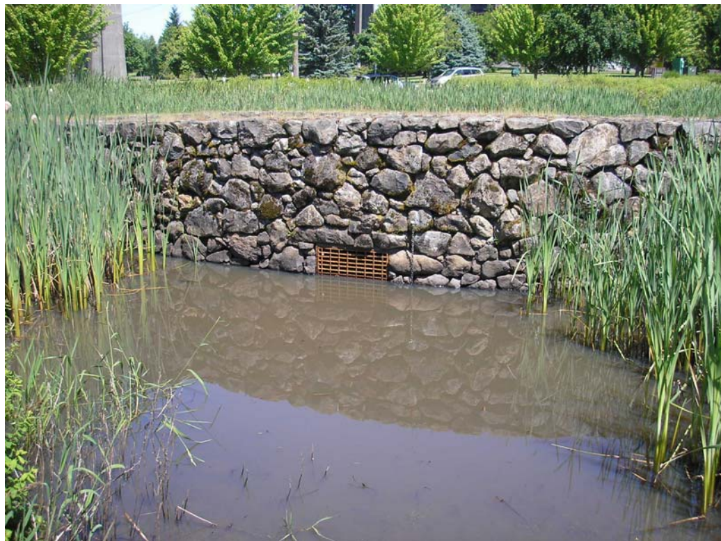
Photograph 2 (June 1, 2007). The solids sample consisted of 3 subsamples collected in the vicinity of the discharge grate.
