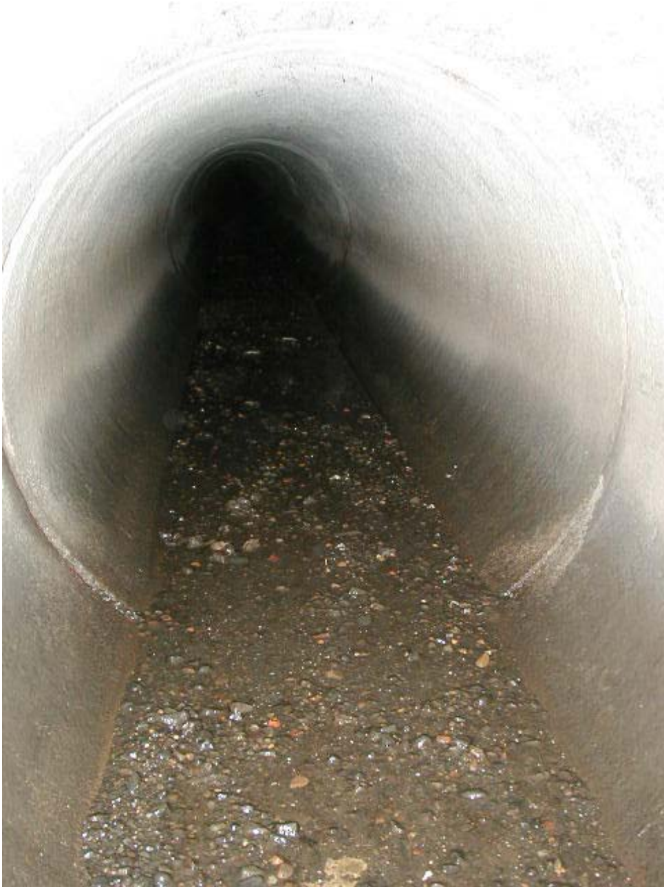
Photo 1 (July, 2005). Inline solids at node AAG648.
