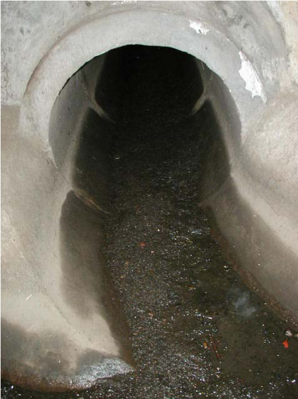
Photo 4 (July, 2005). Inline solids were collected at this location, which is the segment north of node AAG642 and downstream of node AAG649. The western line enters at the bottom left from node AAG648.
