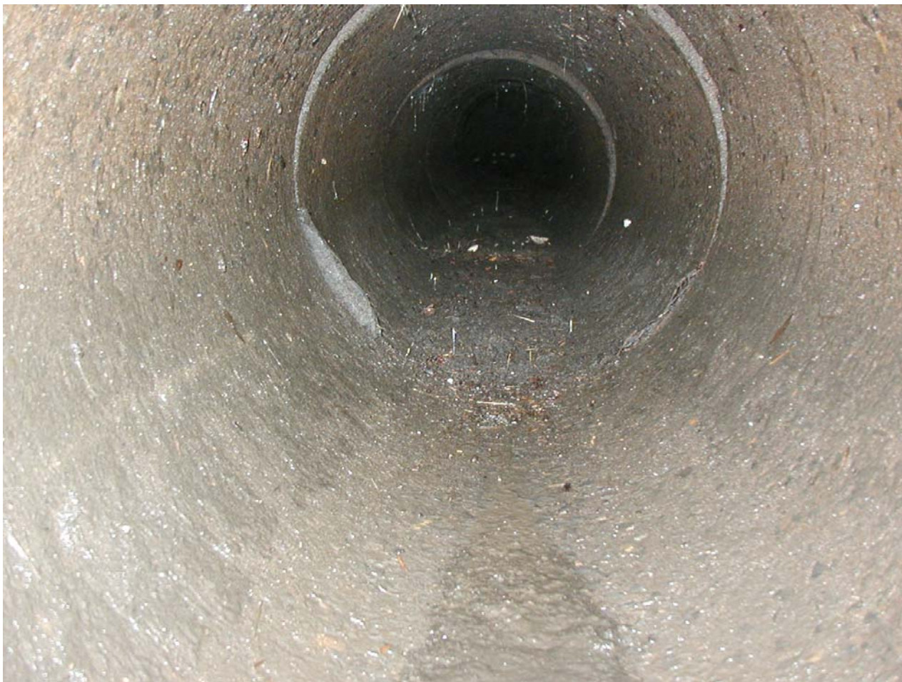
Photo 7 (June 2006). Looking upstream from manhole AAT606 in the 42-inch-diameter line. Inline solids were collected approximately 5 to 10 ft upstream from the manhole.
