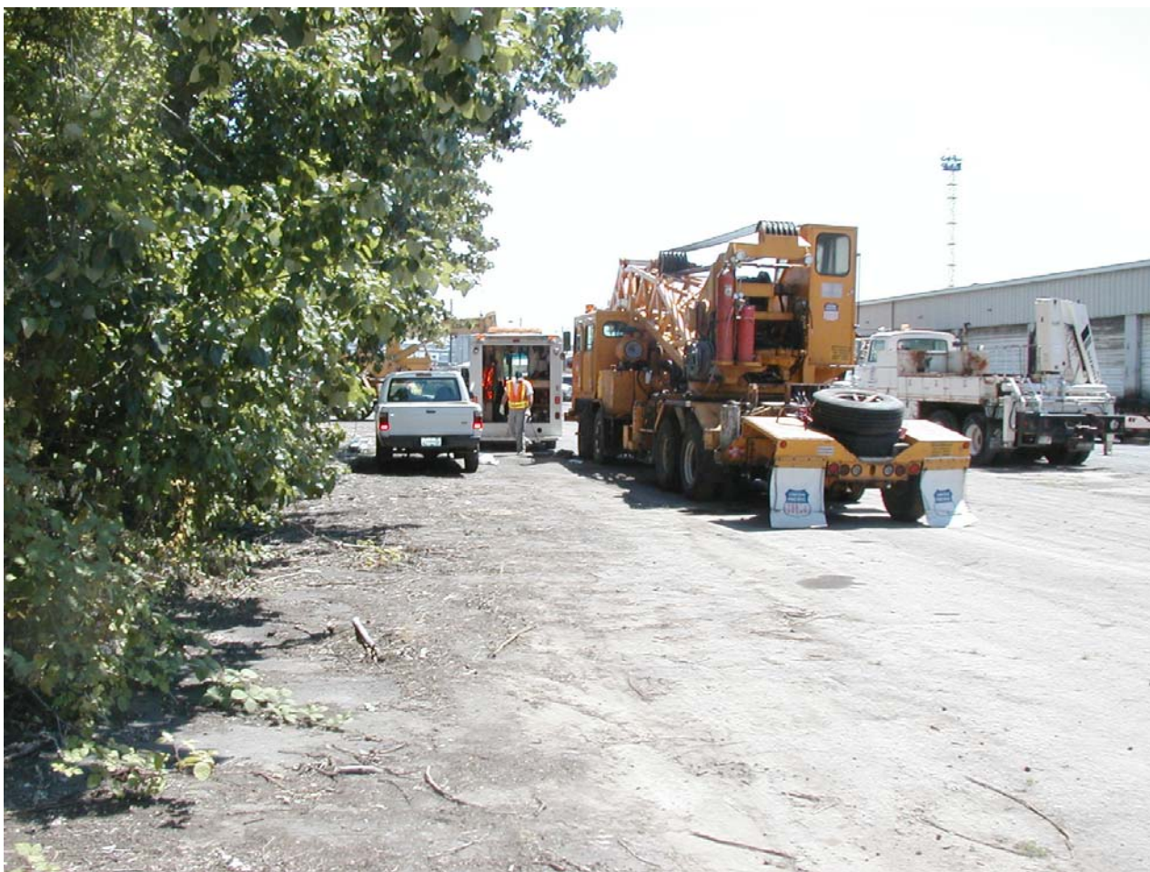
Photo 6 (June 2006). Aboveground location of manhole AAT606 in the UPRR north yard. Two samples were collected at this location, one from the upstream 42-inch-diameter main line and one from an 18-inch-diameter lateral entering from the southwest.
