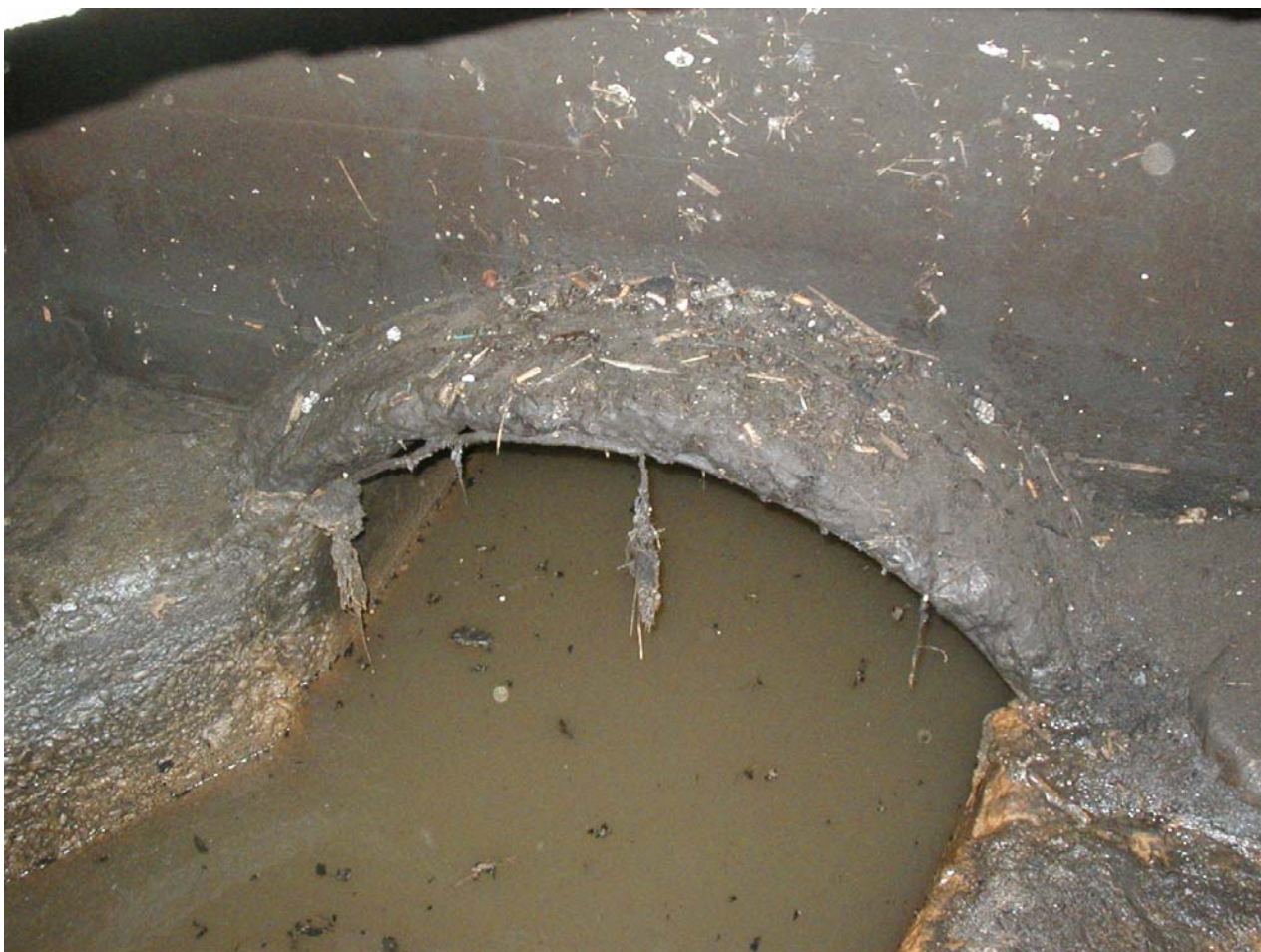
Photo 3 (June 2006). Inside manhole AAQ090. The line was flooded, so a sample was collected from accumulated solids on the ledge above the floor of the manhole (see Photo 4).
