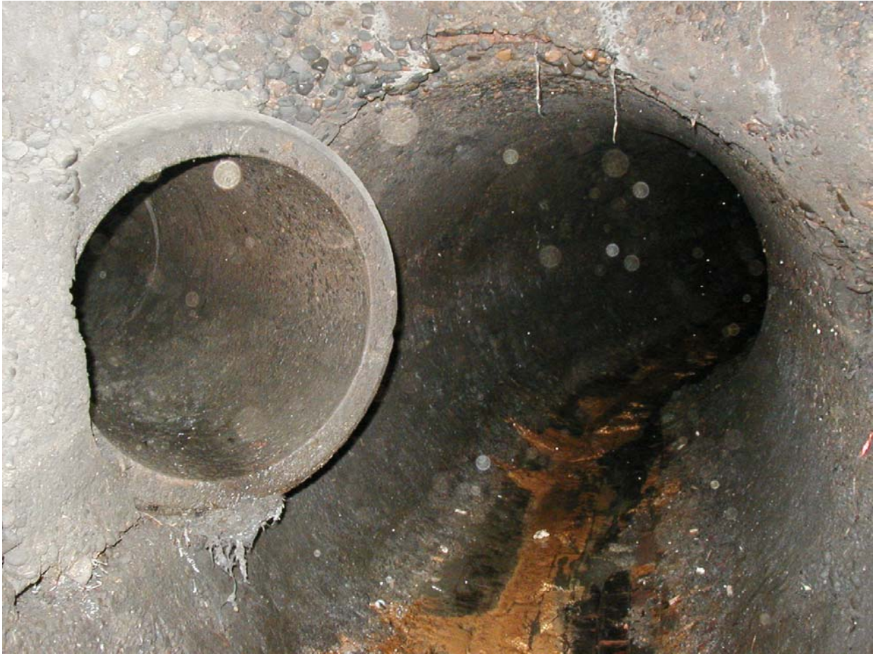
Photo 9 (June 2006). Looking downstream from manhole AAT606, where the 18-inch-diameter lateral enters the manhole from the southwest. Inline solids were collected from the 18-inch line.
