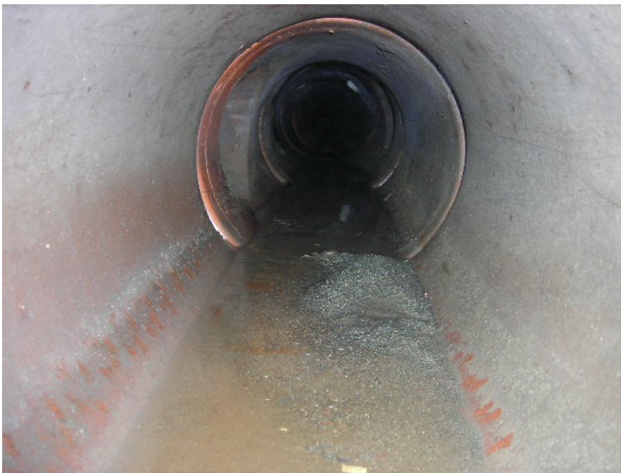
Photo 10 (June 21, 2007). Inline solids sample was collected from the 10-inch-diameter line discharging from manhole ABC318.
