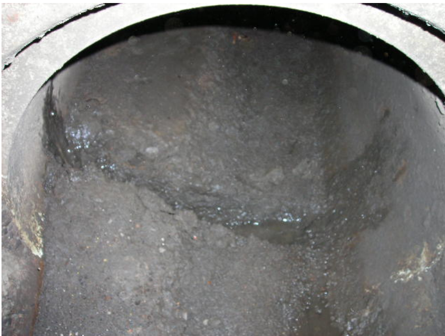
Photo 4 (June 21, 2007). Inline solids were collected from this 24-inch-diameter line discharging to the southwest from manhole AAX693.
