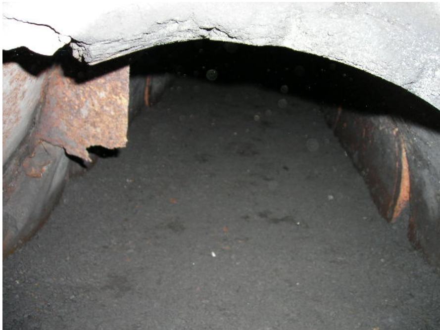
Photo 2 (June 21, 2007). Inline solids were collected from this 22-inch-diameter line discharging to the west from manhole AAX696.
