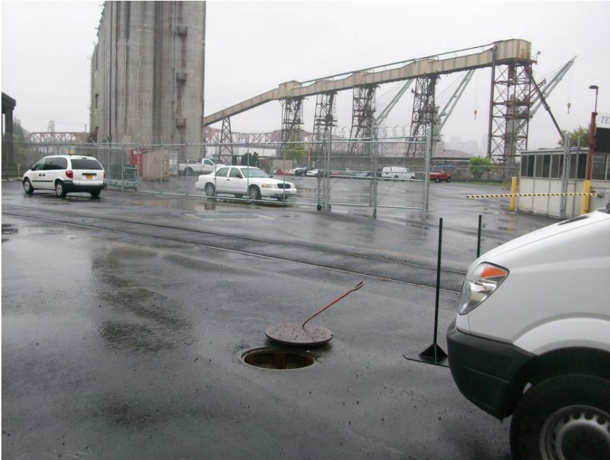
Photo 1 (April 19, 2012). Manhole ANR758 in N. River Street. View is to the northwest.
