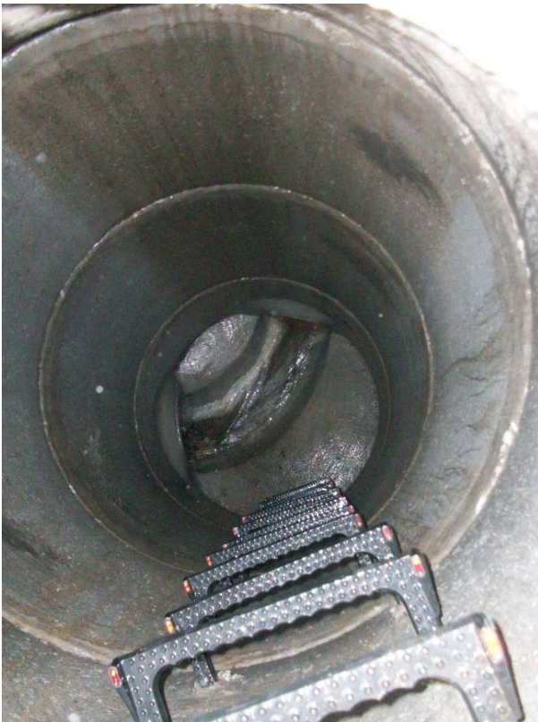
Photo 2 (April 19, 2012). Stormwater flow entering Manhole ANR758 from the northwest.
