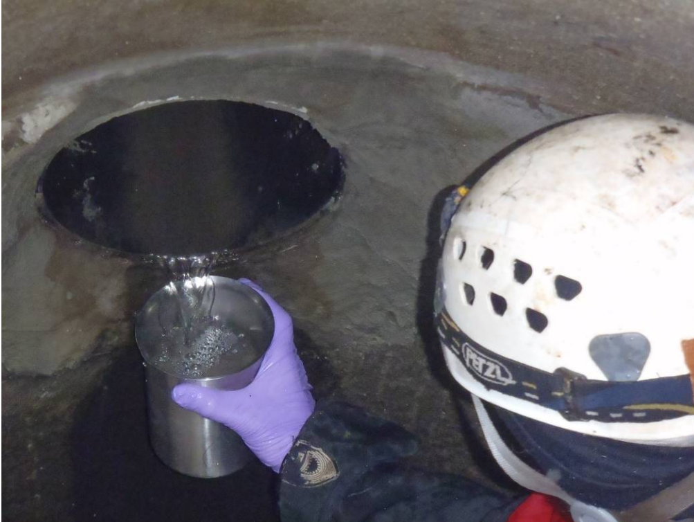
Photo 5 (March 15, 2012). Collecting stormwater sample from 8" line from catch basins APL242, APL243 and APL244.
