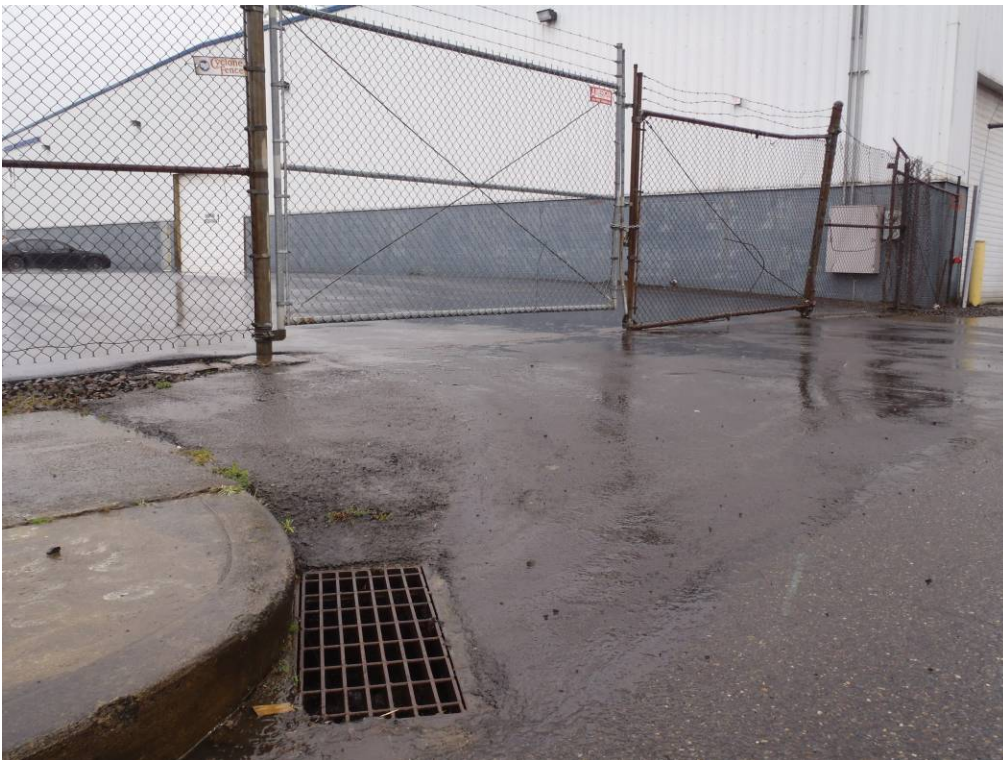
Photo 8 (March 15, 2012). Catch basin APL246 during Basin 44 sampling event. View is to the south-southwest.
