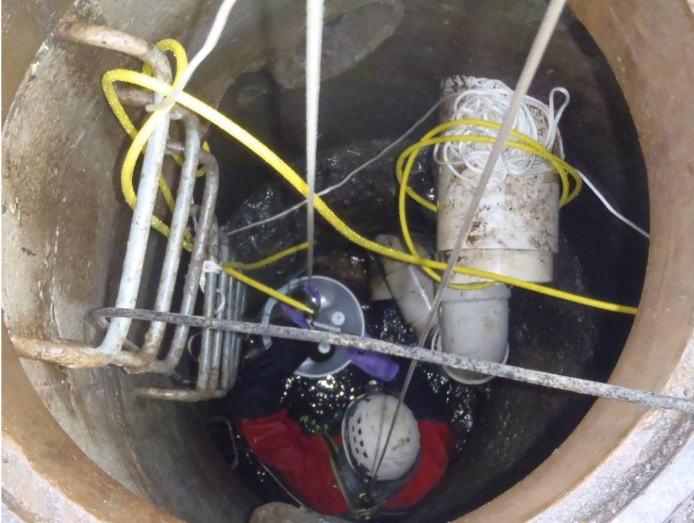
Photo 7 (March 15, 2012). Collecting samples from incoming lines to manhole ABC352.
