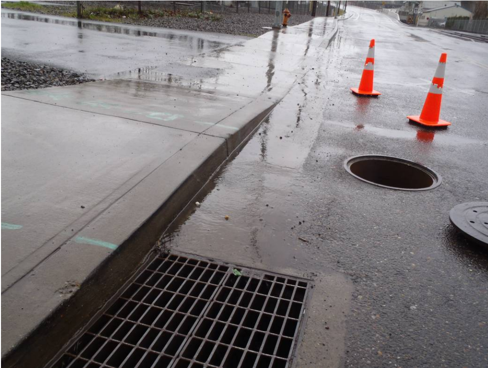
Photo 3 (March 15, 2012). Manhole ABC352 during stormwater sampling event. Catch basin APD919 is visible in foreground. View is to the southeast.
