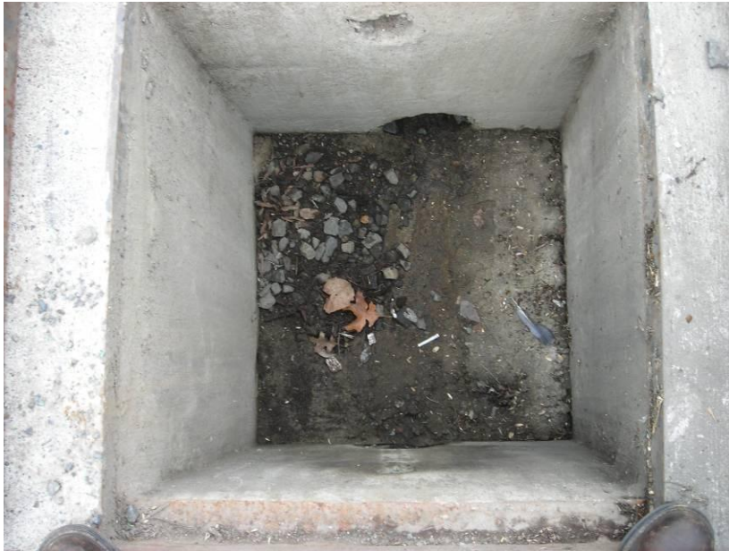
Photo 23 (April 29, 2009). View inside Catch Basin ANE065, showing accumulated solids.
