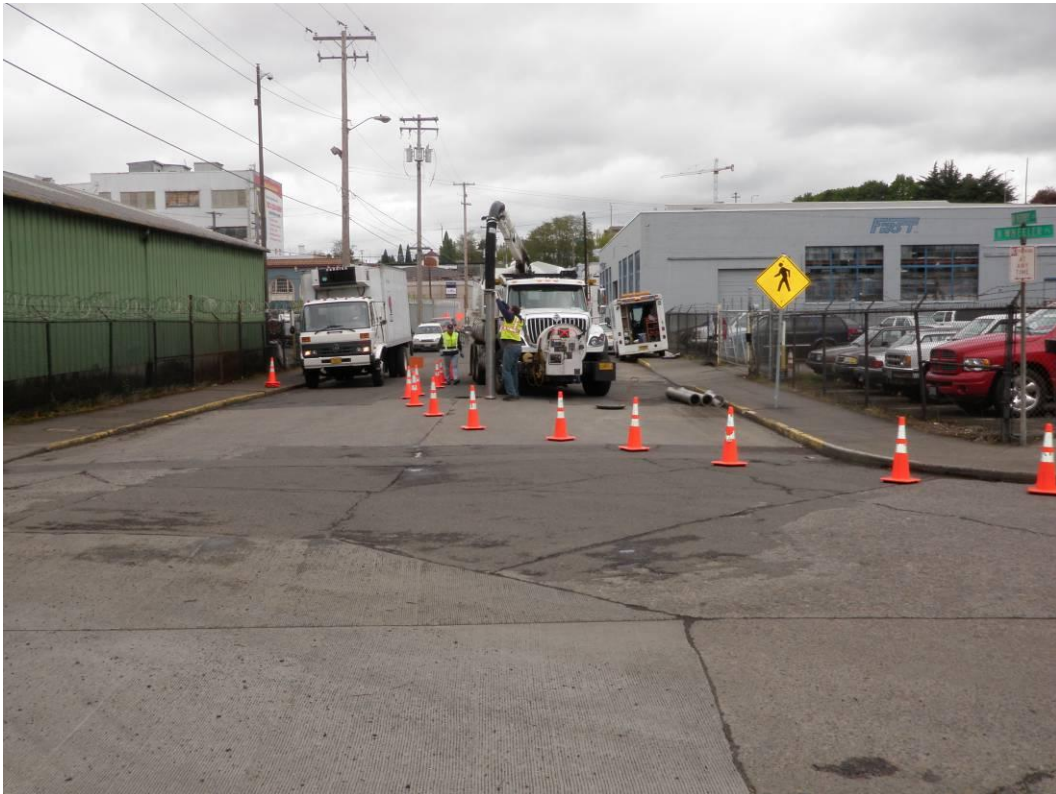
Photo 25 (April 28, 2010). Sampling setup at Manhole ABC539. A vactor truck was utilized to decant stormwater from the manhole.
