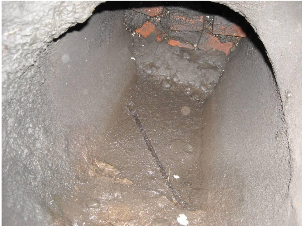
Photo 18 (April 29, 2009). View of solids sampled from the 15-inch line entering Manhole ABC479 from the west.
