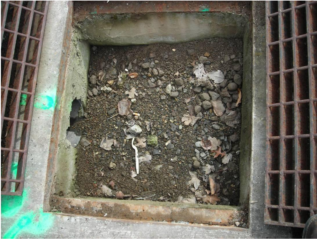
Photo 21 (April 29, 2009). View inside Catch Basin ANE064, showing accumulated solids.
