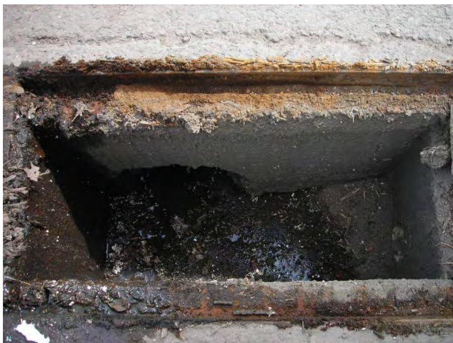
Photo 2. Looking inside catch basin AAT525. These solids were collected for analysis.
