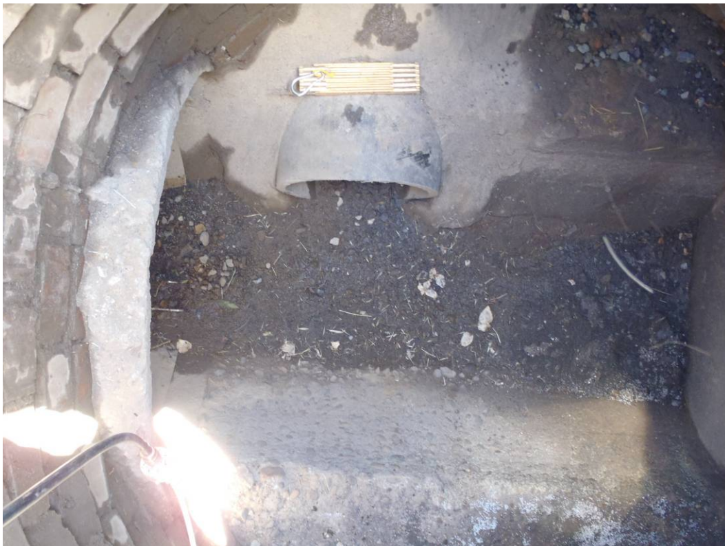
Photo 10 (June 9, 2011). Solids at bottom of Manhole AAX318 before sampling.
