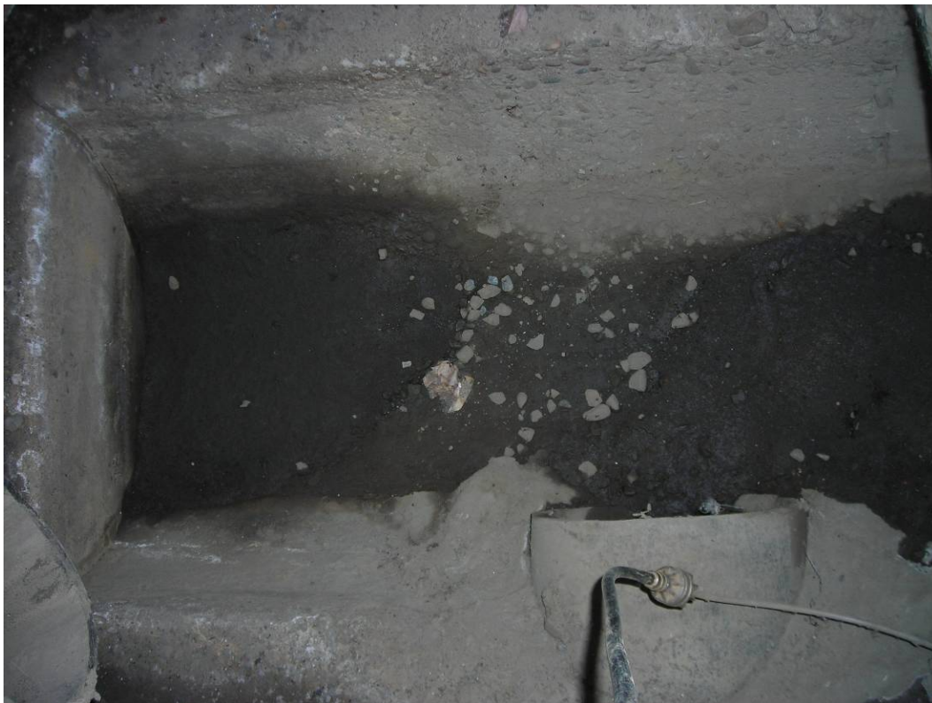
Photo 8 (September 2, 2009). Solids at the bottom of Manhole AAX318.
