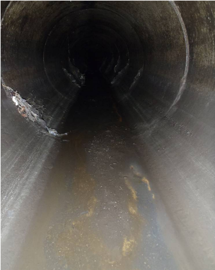
Photo 16 (June 9, 2011). Solids in outgoing 30-inch line from Manhole AAX278 before sampling.
