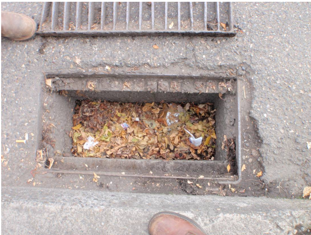
Photo 16 (September 14, 2010). Solids and overlying organic matter and debris in catch basin ANB622 before sampling.
