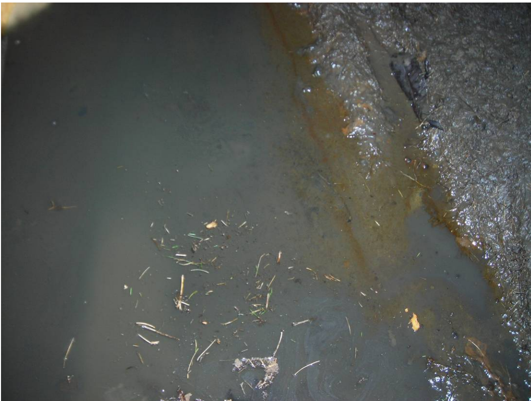
Photo 14 (September 2, 2009). Solids and standing water in Manhole AAX278.
