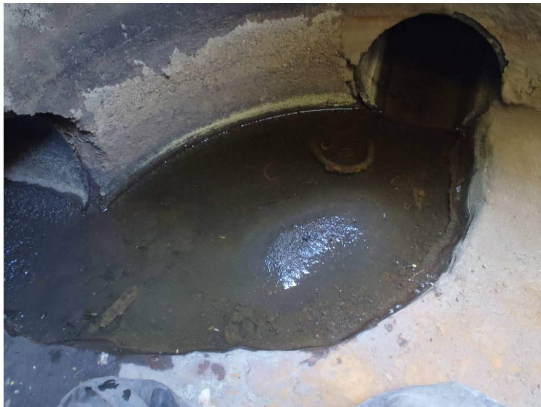
Photo 13 (June 9, 2011). Solids at the bottom of Manhole AAX376 before sampling.
