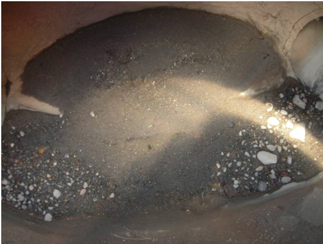
Photo 5 (September 2, 2009). Solids accumulated along west side of Manhole AAX375.
