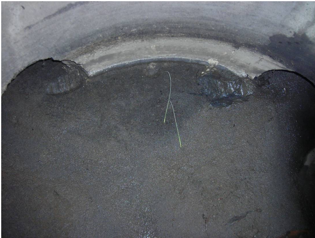
Photo 11 (September 2, 2009). Solids at the bottom of Manhole AAX376.
