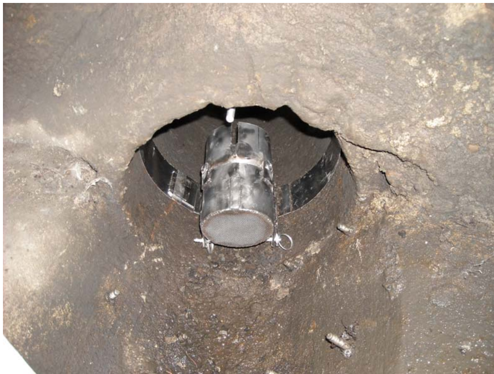
Photo 15 (February 2009). Eastern subbasin sampling location ST1, with installed “SIFT” pilot study sediment trap.
