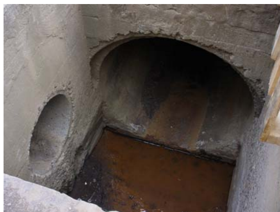
Photos 4-5 (August 2004): Stormwater node AAX316 at Container Management and junction of 18" and 42" stormwater lines at AAX316.
