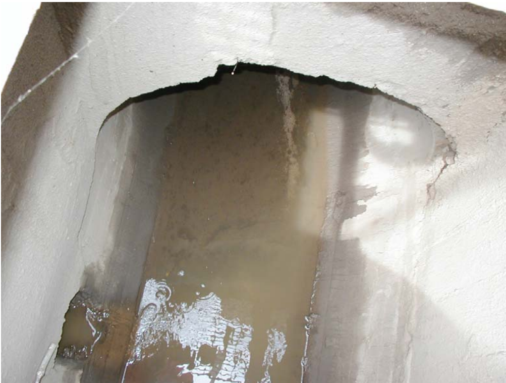
Photo 7 (August 2004): Node AAX281 with Container Management stormwater lateral ANB971 entering from the west during sample collection.
