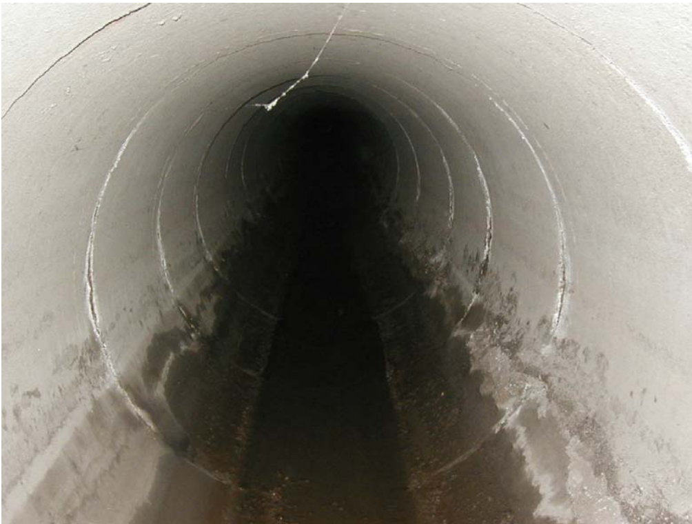
Photo 13 (August 2004): 42" stormwater line downstream of node ANB968.
