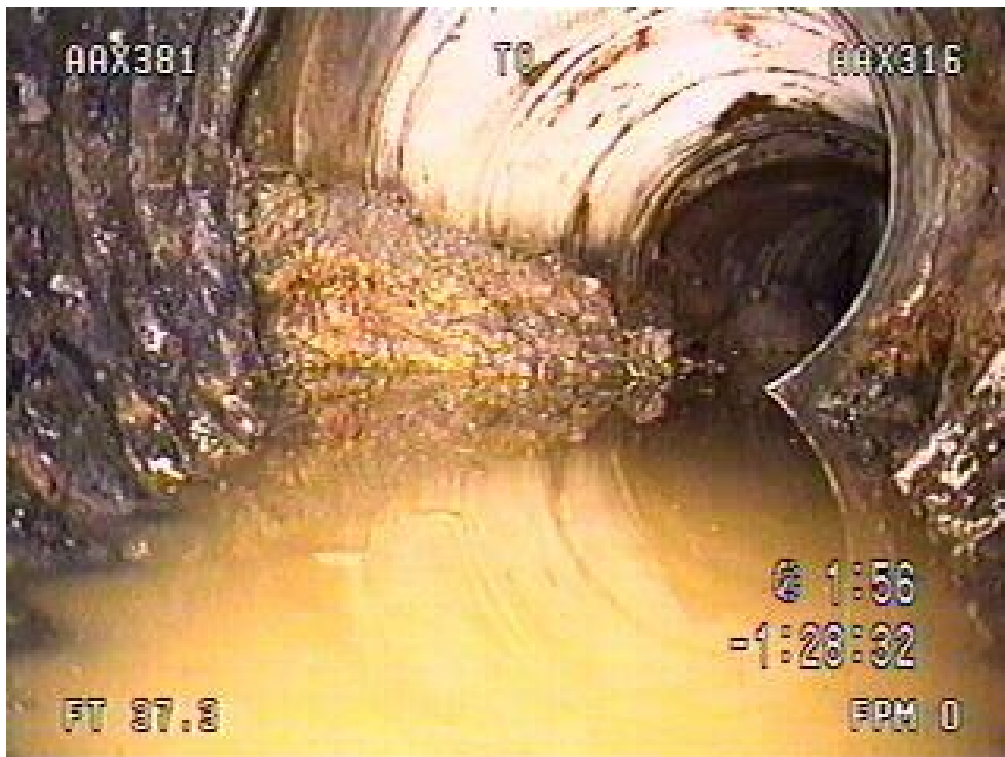
Photo 1 (July 2004): 18" stormwater line - south side of Container Management facility.
