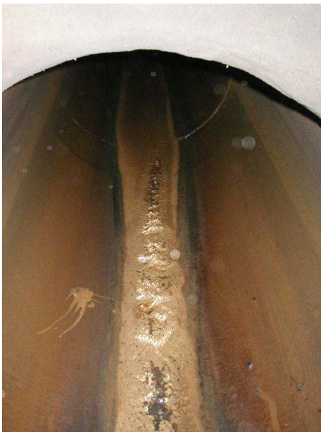
Photo 1 (July, 2005). Inline solids were collected from this location, which is the 48-inch-diameter line discharging from manhole AAX408.
