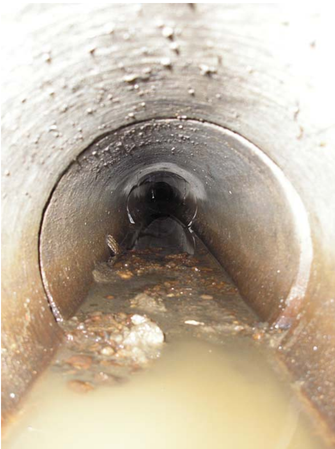
Photo 9 (November, 2005). Inline solids were collected at manhole AAX413 from this 8-inch-diameter line that runs parallel to the main line on Front Avenue. This line is adjacent to the Front Avenue MP property.
