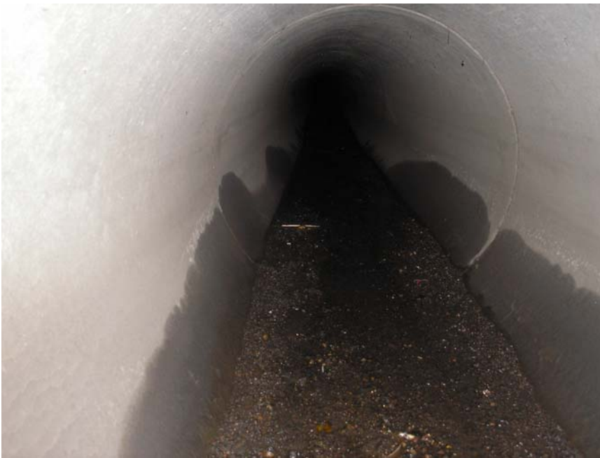
Photo 14 (November, 2005). Inline solids present in the line at manhole AMZ125.
