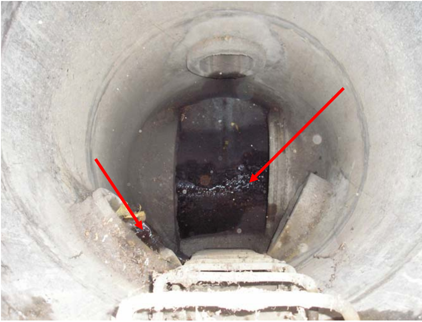
Photo 13 (November, 2005). View looking into manhole AMZ117. Dry-weather flow samples were collected from the main line and the incoming lateral to the left.
