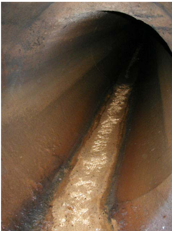
Photo 3 (July, 2005). Inline solids were collected from this 42-inch-diameter line that enters manhole AAX408 from the west.
