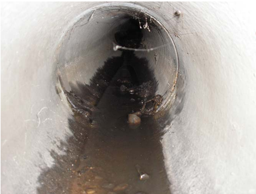
Photo 16 (November, 2005). Inline solids present in one of the lateral lines that enters the main line at manhole AMZ132. Inline solids were collected from both laterals that discharge to the main line and originate at catch basins on either side of Yeon Avenue.
