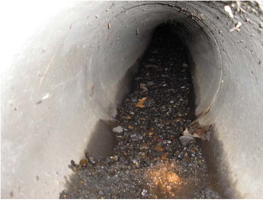
Photo 17 (November, 2005). Inline solids present in the second lateral line that enters the main line at manhole AMZ132.
