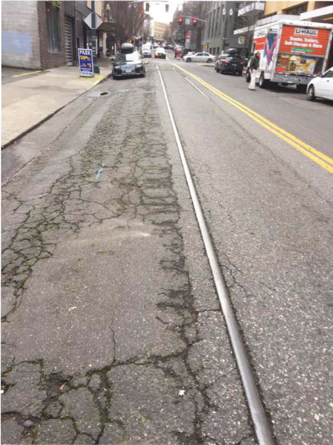
Very poor pavement condition and abandoned rail lines along NW 12 th Avenue project frontage
