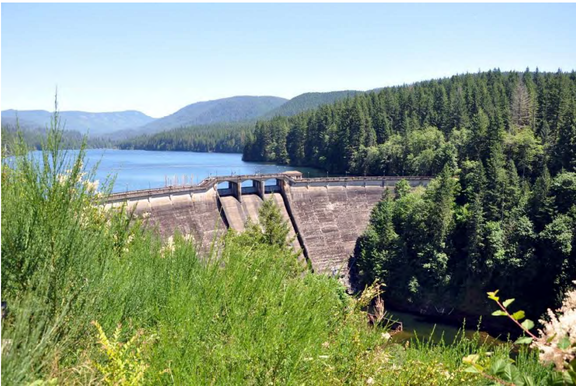
Figure 1.1 Downstream View of Bull Run Dam 1
