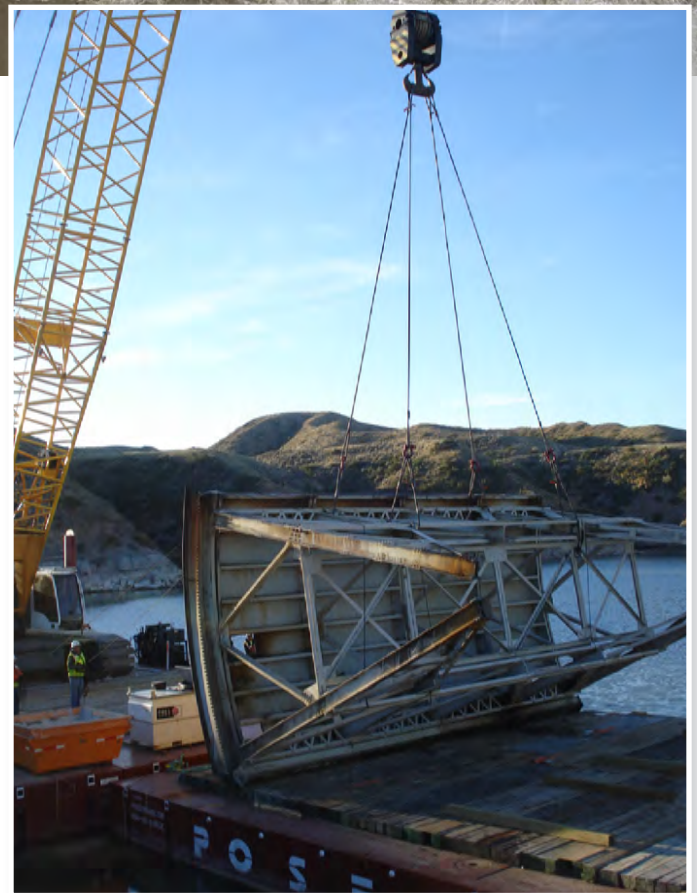
Replacement of 9 radial gates with 36' x 26' vertical roller gates (60kips each)
