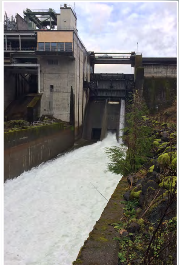
McMillen Jacobs is building a numerical and physical model of the sluice gates to develop modifications and alternatives to the sluice intake, gate type, and exit
