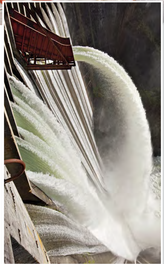
Replacement of 22 gates with 12 vertical roller gates (13' x 20')
