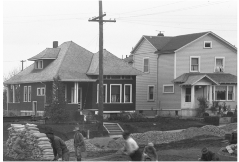
Although outside of the Historic District, this 1926 photo of the Ross Island Bridge under construction shows representative examples of the craftsman/bungalow styles found in South Portland. Image courtesy Portland City Archives, A2009-009.486.
