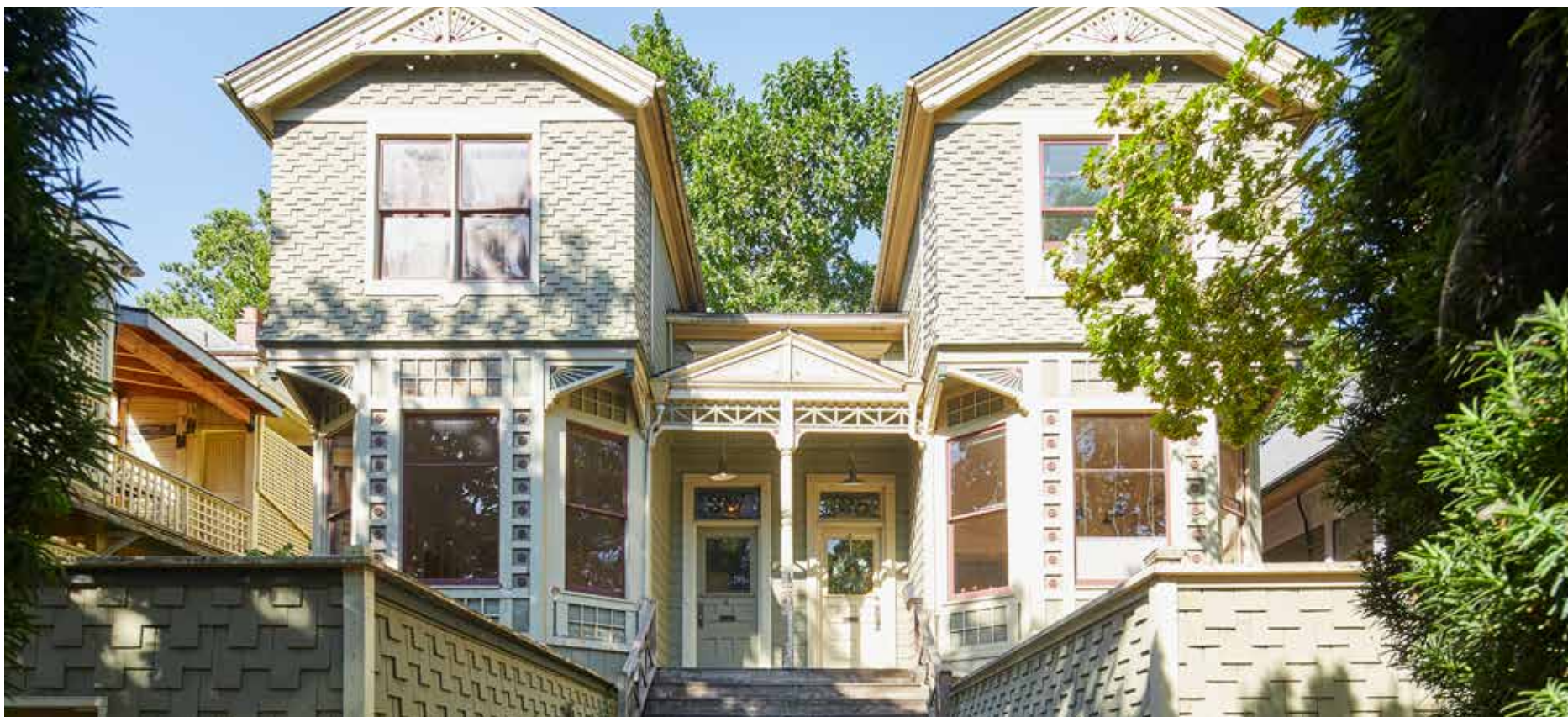
An 1894 plex on S Water Avenue demonstrating a high degree of preservation of street-facing character-defining features and materials.
