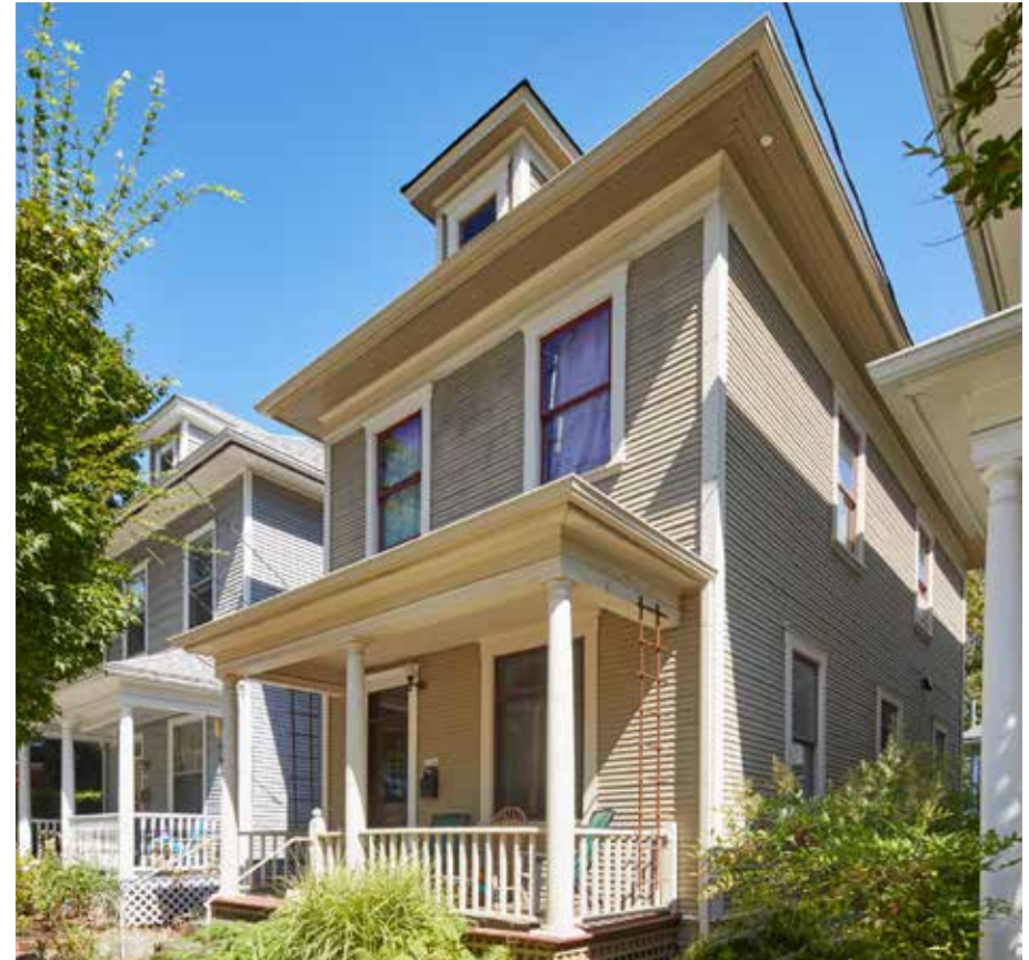
Relating window patterns, projecting eaves, and roof forms from nearby contributing buildings of a similar typology into the design of new construction.
