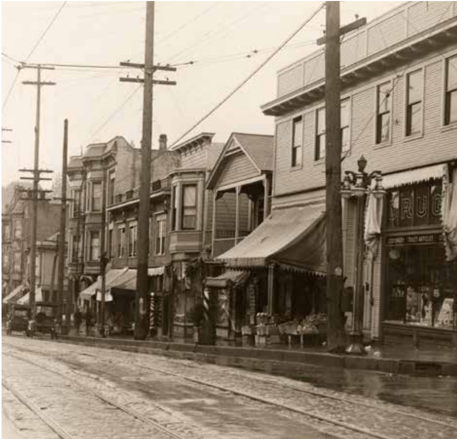
Selecting the mixed-use building typology for sites along the historic streetcar route.
