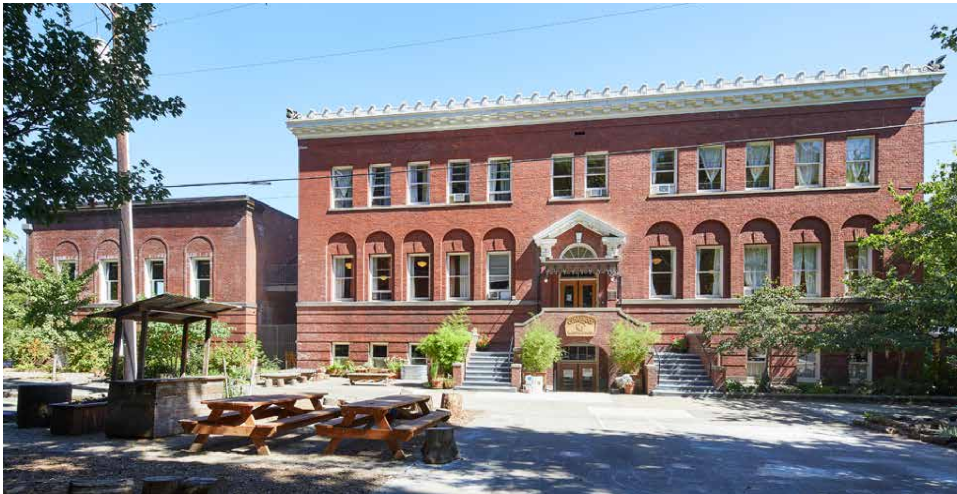
The 1926 addition (at left) to the Neighborhood House complemented the style and proportions of the original 1910 building.
