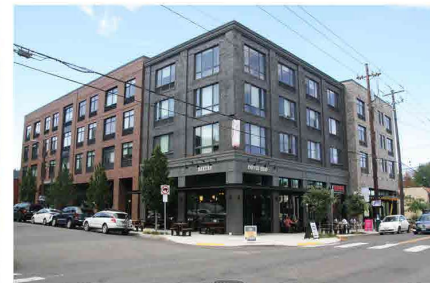
George Besaw Apartments, Portland
